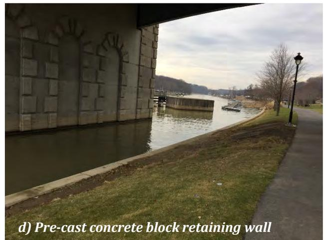
*d) Pre-cast concrete block retaining wall*
