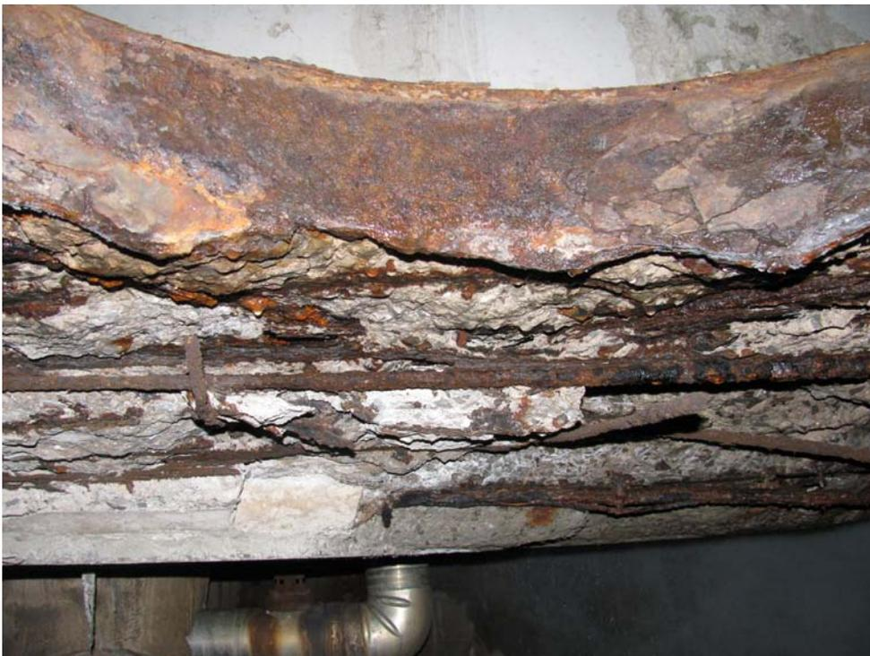
48. Level C: Utility Tunnel Roof Slab Deterioration
