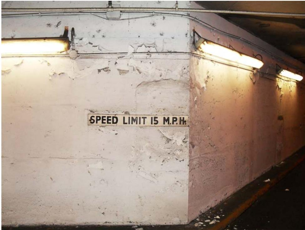
34. Level C: Typical Wall Coating Condition
