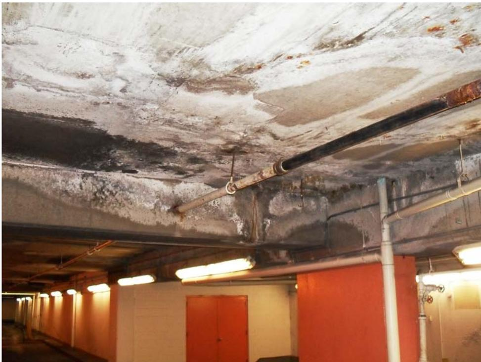
15. Level B: Ceiling Deterioration
