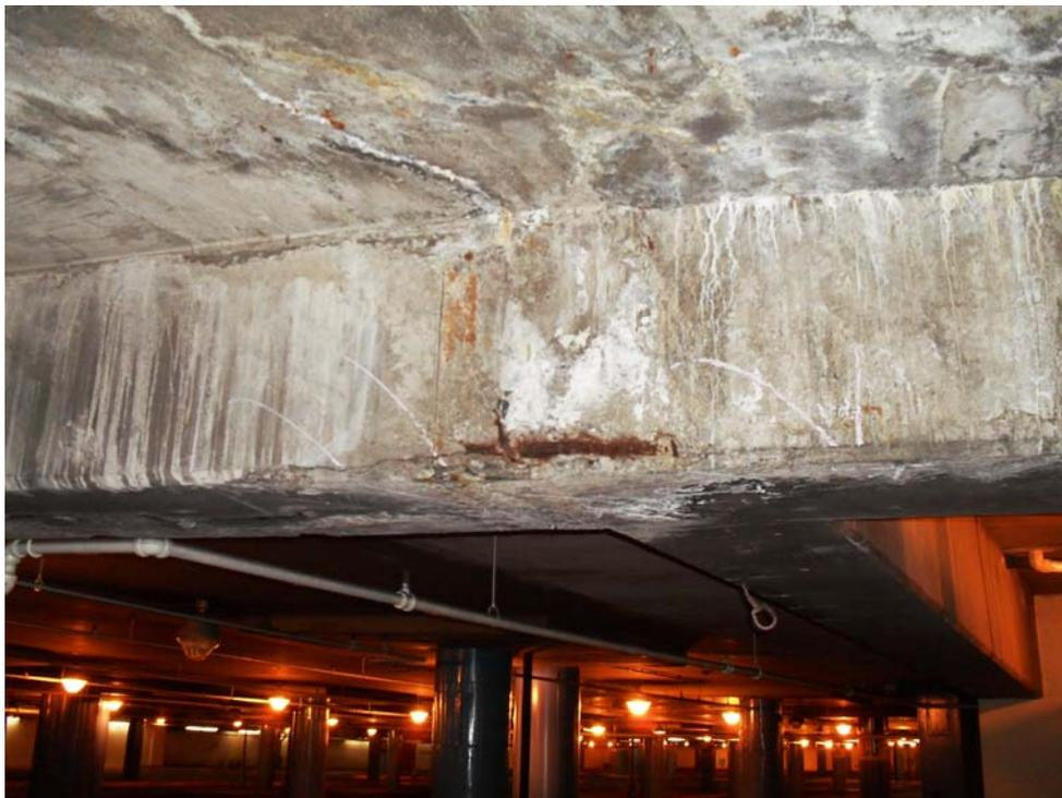
20. Level C: Ceiling and Beam Deterioration
