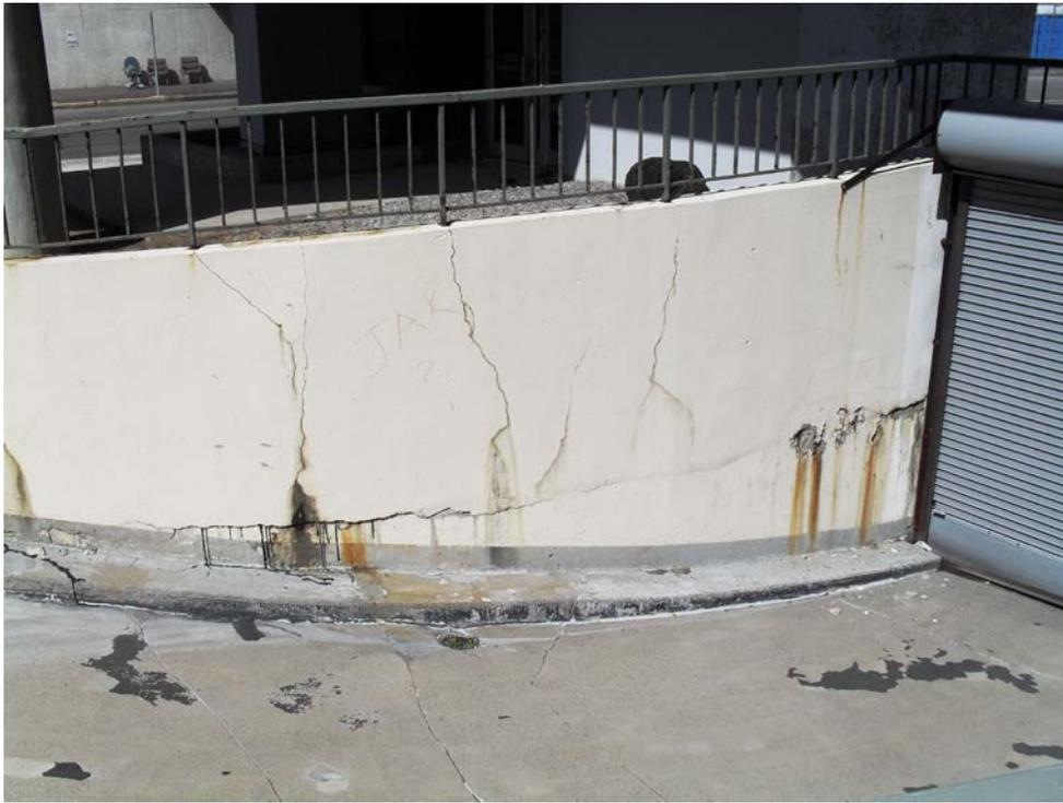
45. Broad Street Exit: Retaining Wall Cracks at Railing Posts
