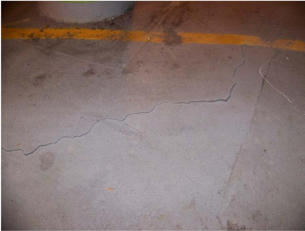
3. Level A: Crack in Traffic Membrane
