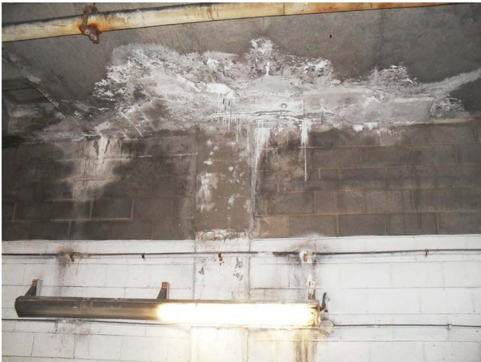
44. Exit to Court Street: Ceiling Deterioration and Column Cracking
