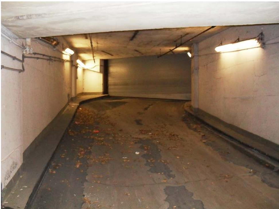
46. Broad Street Exit: Worn Traffic Membrane and Transverse Floor Crack
