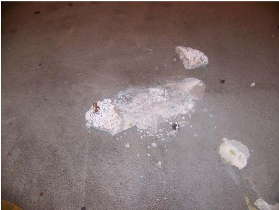
4. Level A: Debonding in Traffic Membrane & Deterioration in Concrete Overlay
