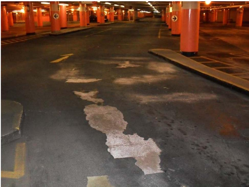
6. Level B: Transverse Crack in Exposed Concrete Overlay
