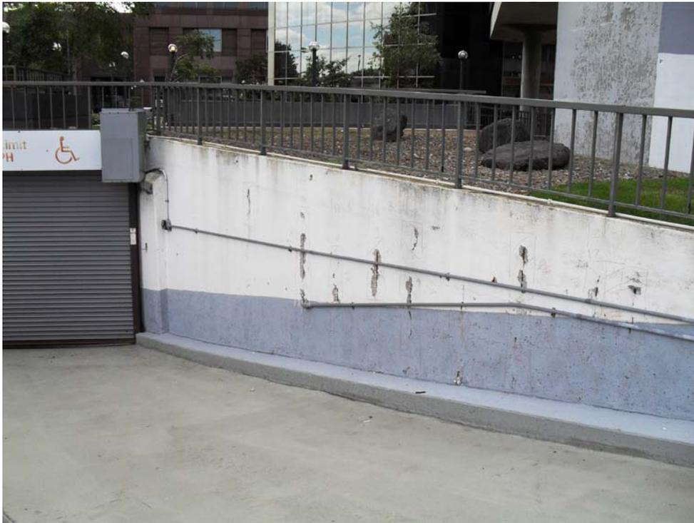
43. Broad Street Entry: Retaining Wall Isolated Spalls
