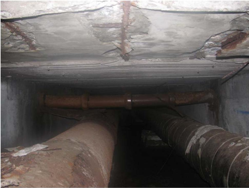
47. Level C: Utility Tunnel Roof Slab Deterioration
