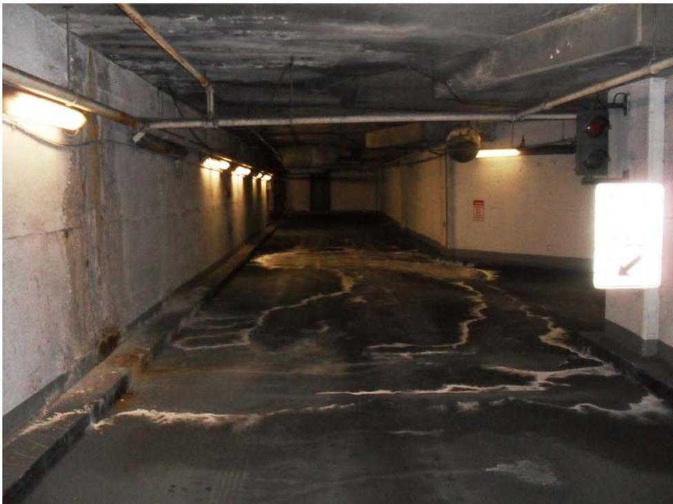
29. Level A: Exit to Court Street Efflorescence Buildup on Floor
