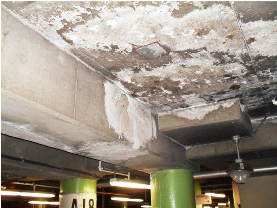
10. Level A: Ceiling and Beam Deterioration
