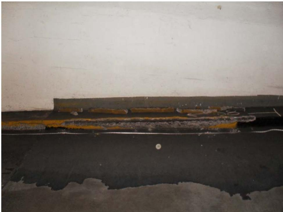
35. Level B: Curb Spall with Exposed Rebar
