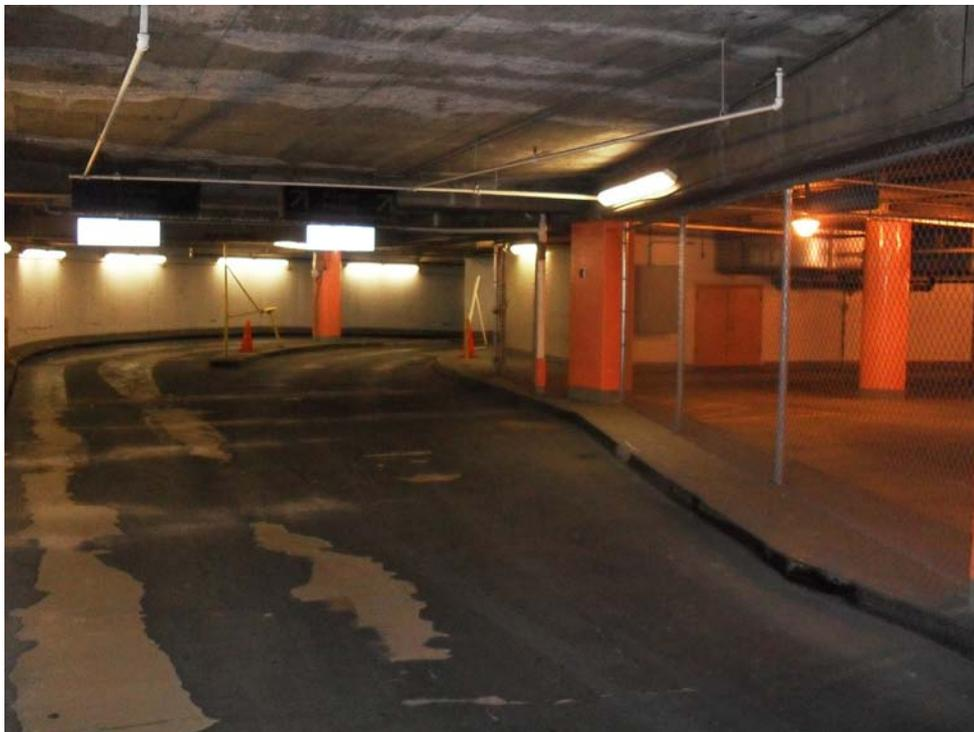
8. Level B: Worn Traffic Membrane in Recirculation Aisle
