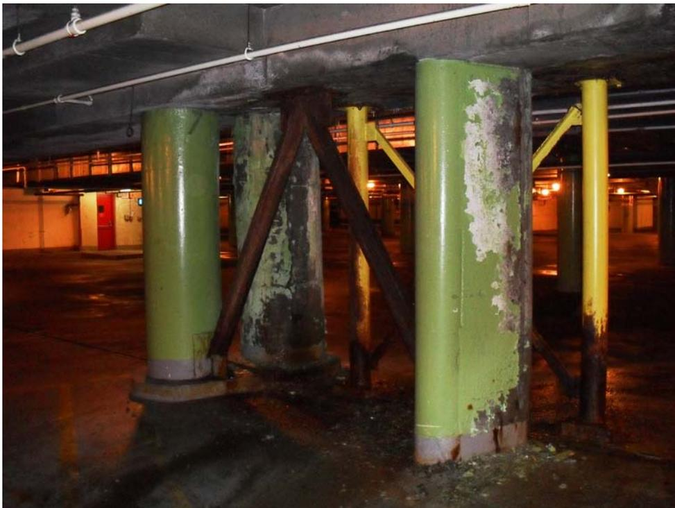
24. Level A: Columns 5-H and 5.4-H.1 Deterioration at Leaking Expansion Joint
