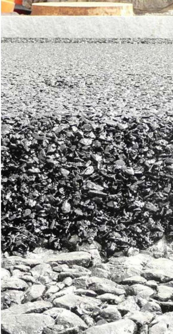
***Porous asphalt cross section,
