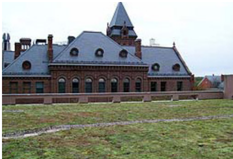
City Hall Green Roof
