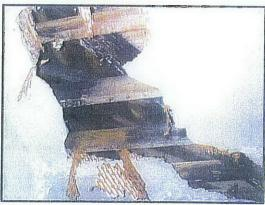
is approximately 220 ft<sup>2</sup> of mold growth estimated in the building. The scope of mold impacted building materials includes (but is not limited to) plaster, roof framing, wooden wooden doors and wooden window/door The concentration of airborne mold spores is 13,455 spores/m<sup>3</sup>.
