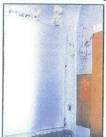
3" floor slab has heaved in several locations. An inspection of the roof framing illustrated the growth of wood rot fungi and deteriorated wooden members due to chronic roof leaks. The roof on the east side of the structure has failed and is supported to prevent collapse. There
