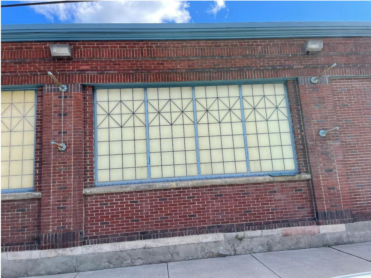
*West wall, horizontal mortar joints in brick masonry have failed as brick drops with sagging steel lintels.*
