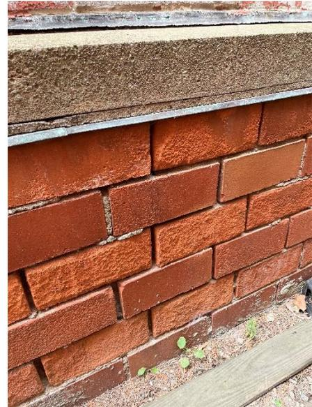
*East wall with faux-brick panels over precast concrete, over structural clay-tile masonry.*
