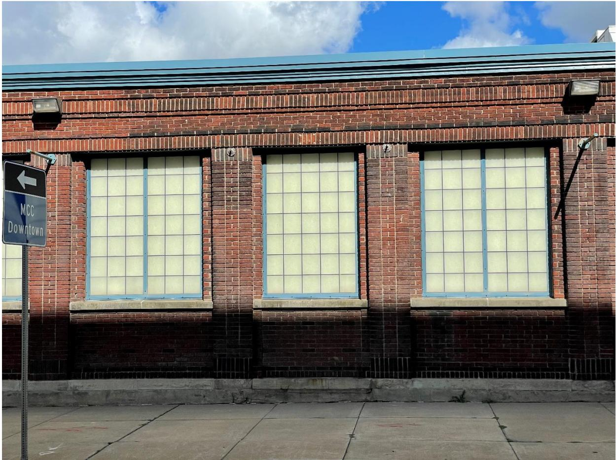
*South wall, in need of foundation parging, brick masonry repointing, and re-sealing window perimeters.*
