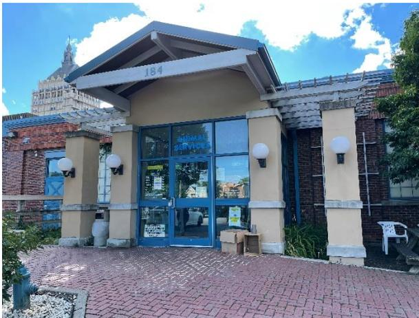
*Wood entry trellis and parged masonry columns.*
