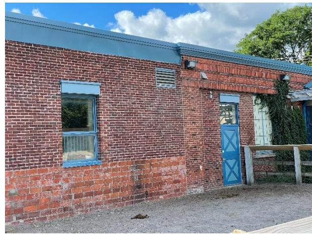
*Cracked and spalled clay-tile masonry water-table.*
