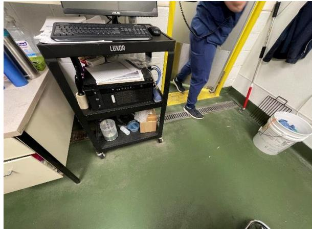
Surgery: Open shelving, trench drains, porous and friable ceilings, and HVAC air flow are not conducive to infection control.
