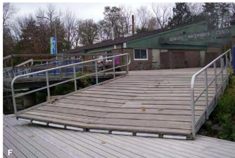
A. Rower Docks, looking North      B. Rower Docks, looking South      C. "Strong-Arm" Dock Mooring System      D. Steel Pipe Piles with Roller Guides      E. Accessible Gangway to rower docks      F. Rower Access Gangway; note uneven toe, and lack of hinge plate (tripping hazards)
