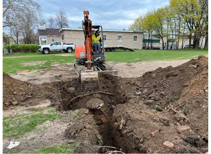
**Photo No. 2** Start of UST Excavation
