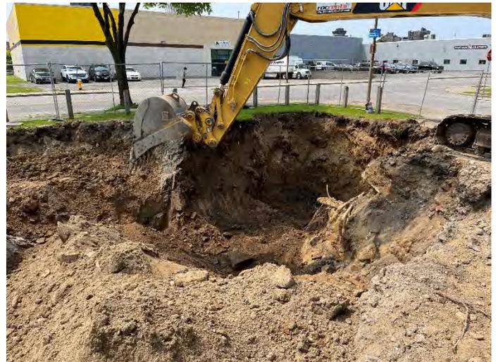
Photo No. 28 Excavation Expansion to Address Impacted Soils
