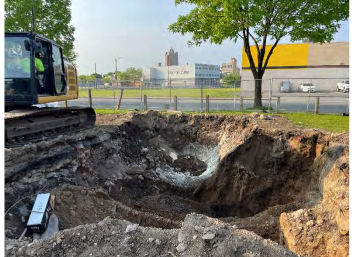
Photo No. 26 ORC Powder Installed Beneath Former UST-05, 06 & 07
