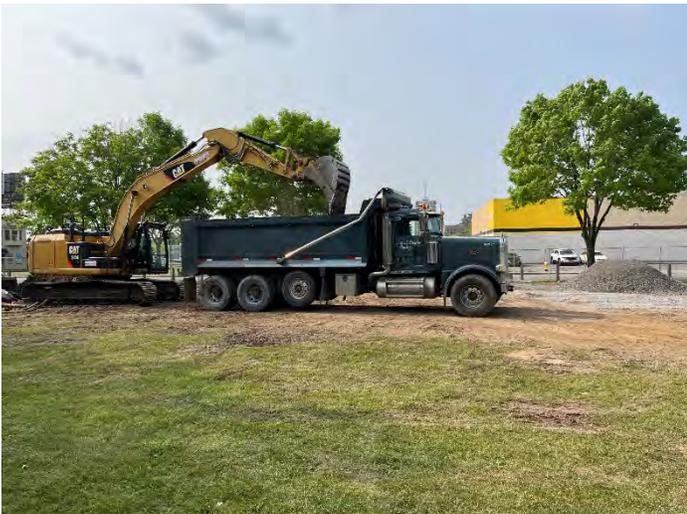
**Photo No. 33** Loading Excess Overburden Soils for Disposal
