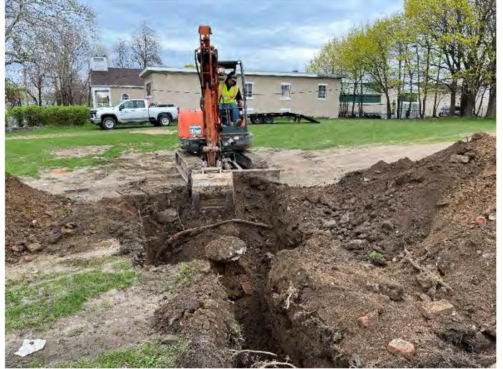
**Photo No. 2** Fill-port of UST-02 Identified During Excavation
