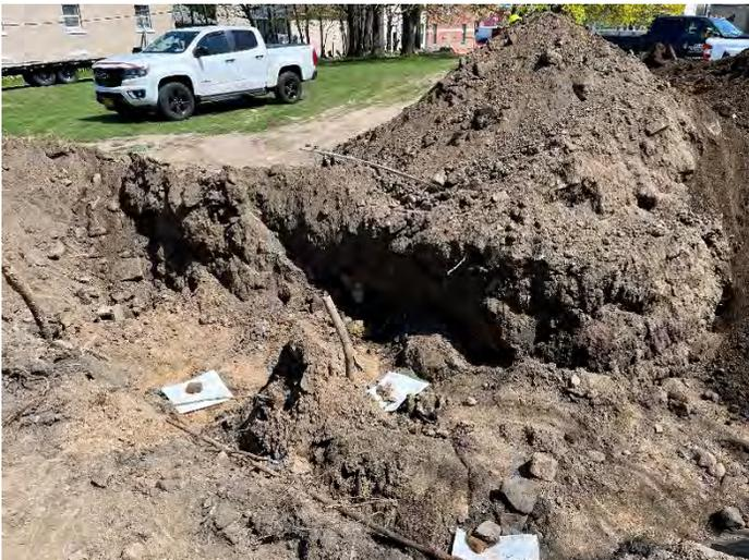
**Photo No. 3** Sorbent Pads Covering UST-02 through 04 Access Points
