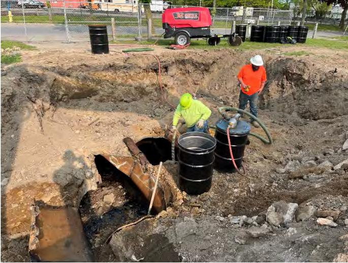
Photo No. 13 Sludge Extraction from UST-03 & 04
