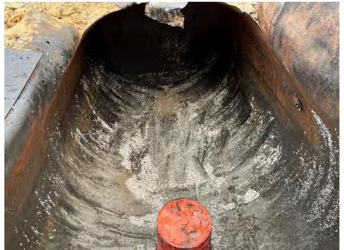
Photo No. 16 UST-03 After Interior Cleaning
