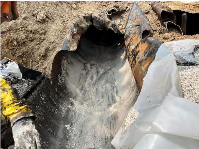
Photo No. 15 UST-04 After Interior Cleaning
