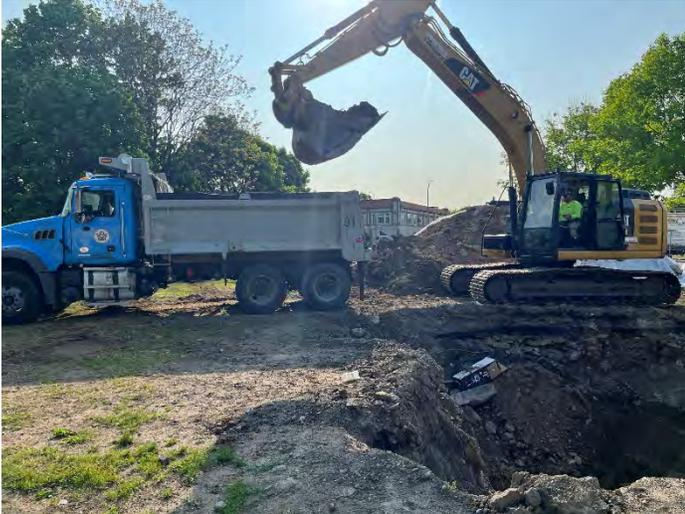
Photo No. 25 Live Loading of Soils from Beneath the Former USTs
