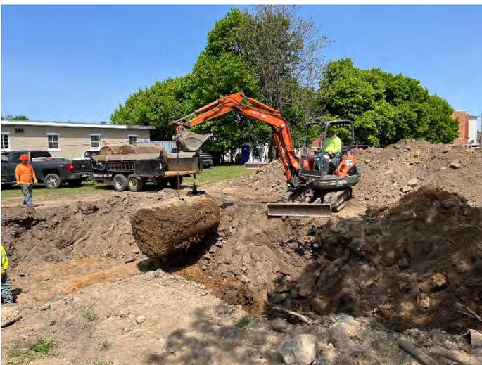
Photo No. 11 Removal of UST-05 (UST-06 & 07 Pictured on Trailer)
