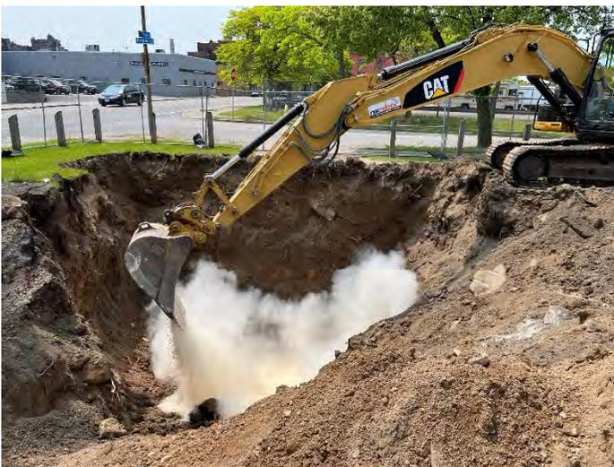
Photo No. 29 ORC Installed in Southwest Corner of the Excavation
