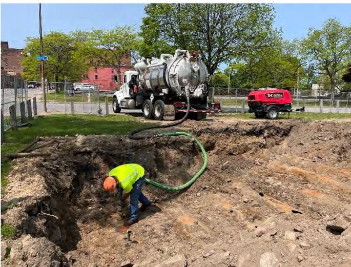
**Photo No. 5** Extraction of Water from Within UST-07
