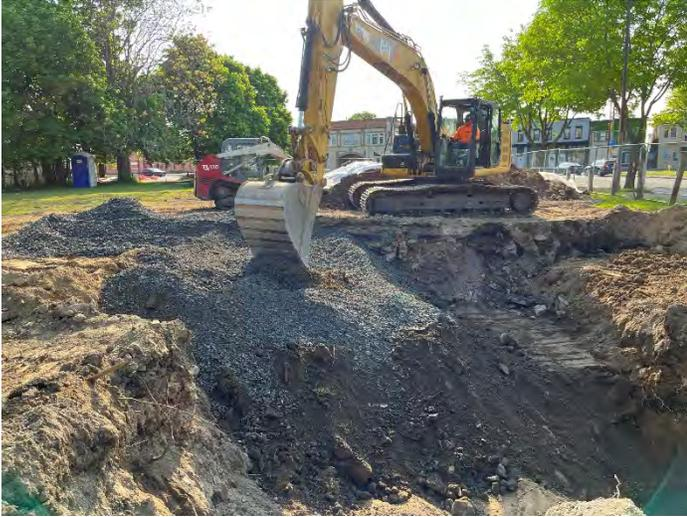
**Photo No. 31** Excavation Backfill and Surface Restoration Process
