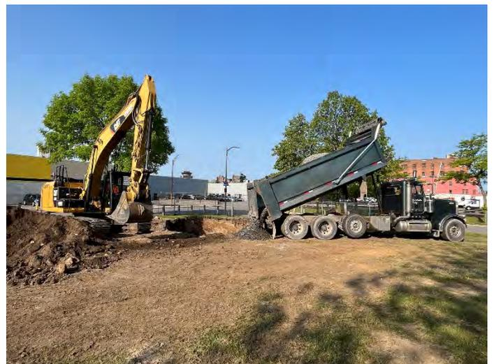
Photo No. 30 Stone Imported for Surface Restoration During Backfill
