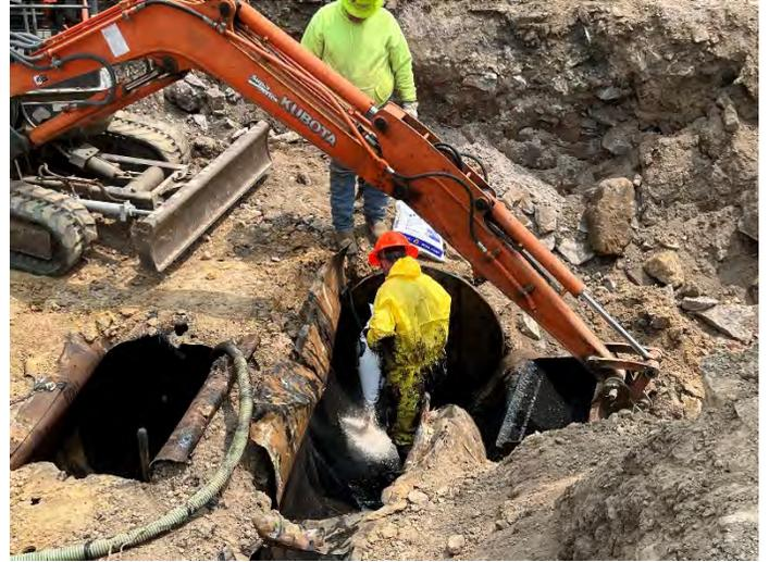
Photo No. 14 Interior Cleaning of UST-04 (UST-03 Pictured Left)
