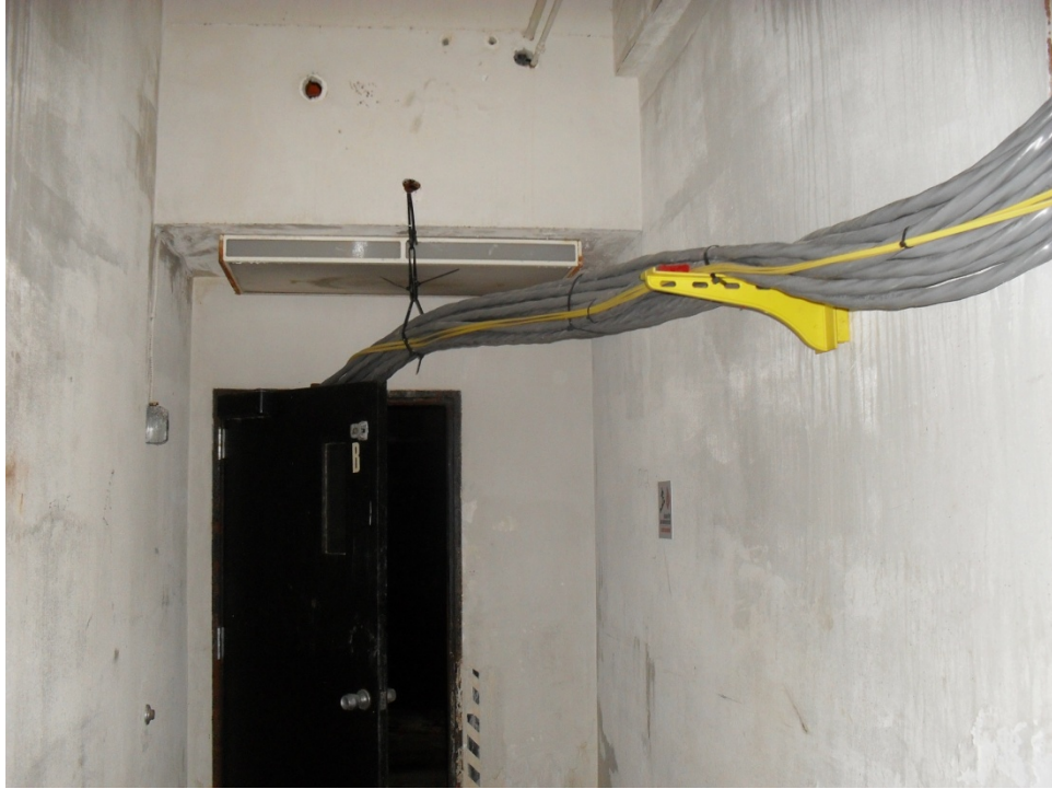
E-5: TEMPORARY POWER DISTRIBUTION CABLING IN STAIR TOWER
