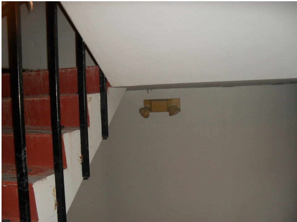
E-8: TYPICAL ABANDONED IN PLACE LUMINAIRE
