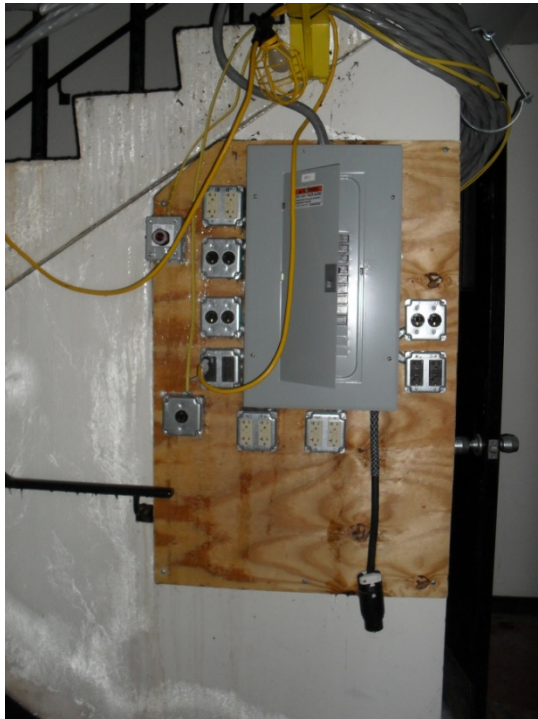
E-6: TEMPORARY POWER DISTRIBUTION PANEL IN STAIR TOWER
