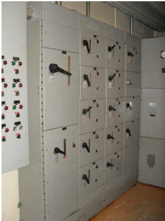
E-4: ABANDONED MOTOR CONTROL CENTER
