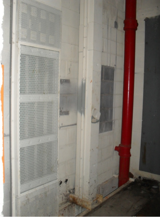
E-7: VERTICAL SECTIONS OF BUSS DUCT IN STACKED CLOSETS
