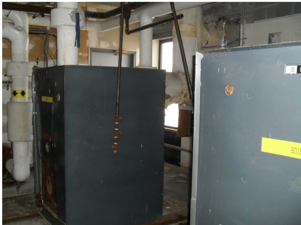
Abandoned boilers in penthouse mechanical space
