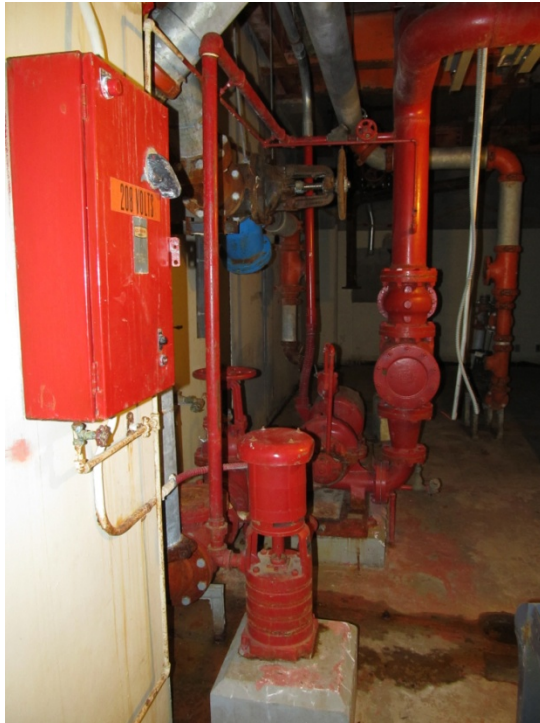
Fire Pump Station in Basement
