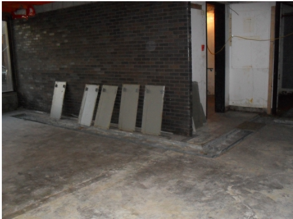
E-12: IN-FLOOR RACEWAY SYSTEM AND COVERS
