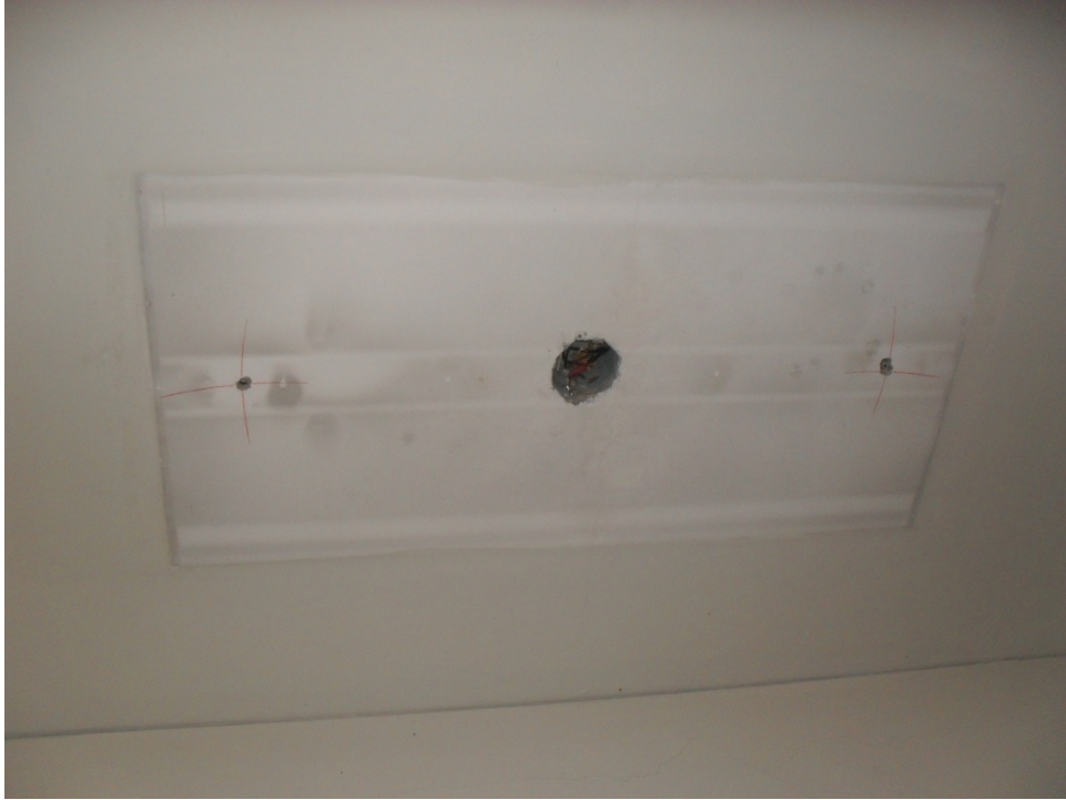
E-9: LUMINAIRE RACEWAY RECESSED IN CONCRETE STAIR TOWER
