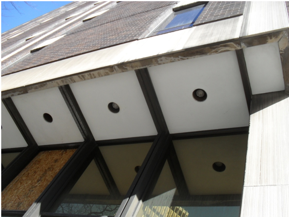
E-10: SOFFIT MOUNTED LIGHTING AT BUILDING ENTRANCE
