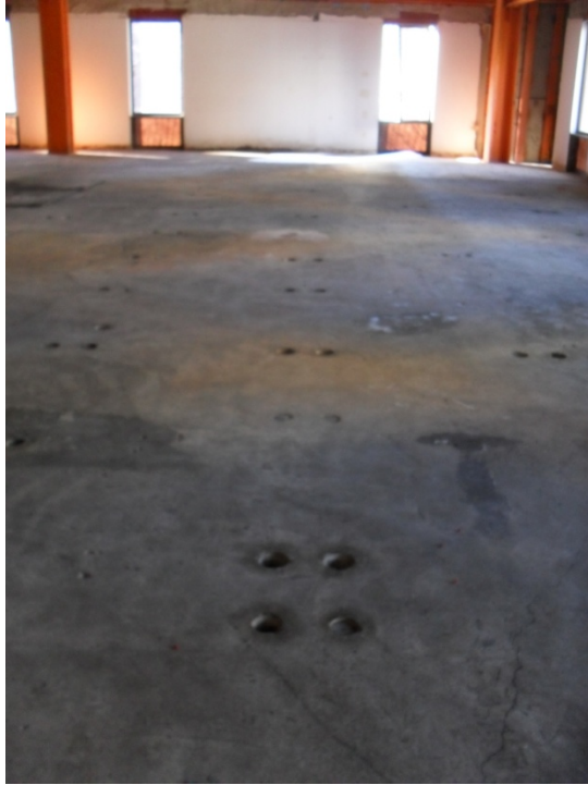
E-15: IN-FLOOR RACEWAY PENETRATIONS AND THROUGH-FLOOR PENETRATIONS
