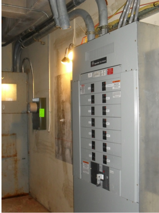
E-3: TEMPORARY SERVICE ENTRANCE SWITCHBOARD
