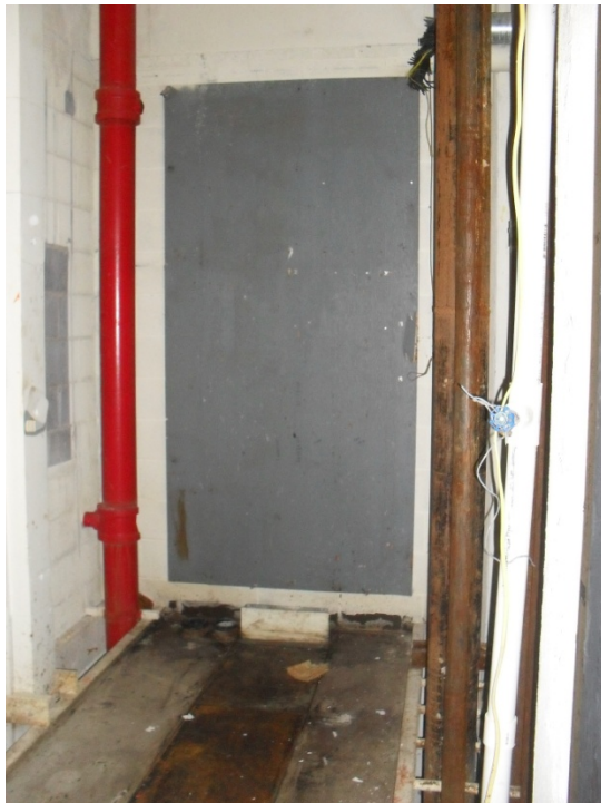
E-14: IN-FLOOR RACEWAY IN STACKED CLOSET AND TELECOMMUNICATIONS BACKBOARD
