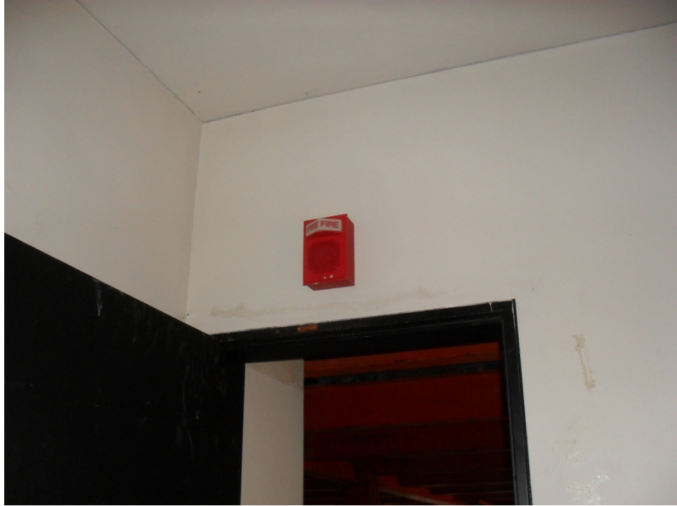
E-11: TYPICAL ABANDONED IN PLACE FIRE ALARM DEVICE
