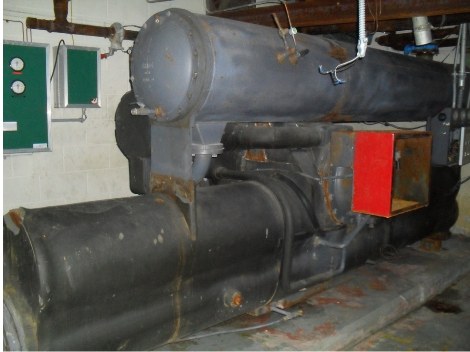
Abandoned Centrifugal Chiller located in basement
