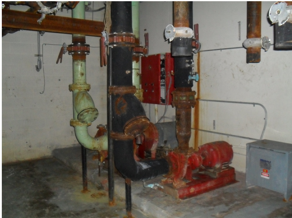
Abandoned chilled water and condenser water pumps
