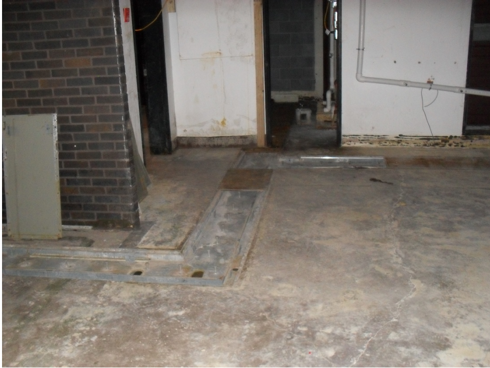
E-13: IN-FLOOR RACEWAY SYSTEM ENTERING STACKED CLOSET
