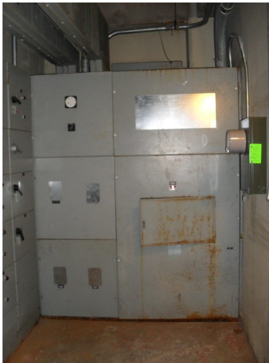
E-2: ABANDONED SERVICE ENTRANCE SWITCHBOARD
