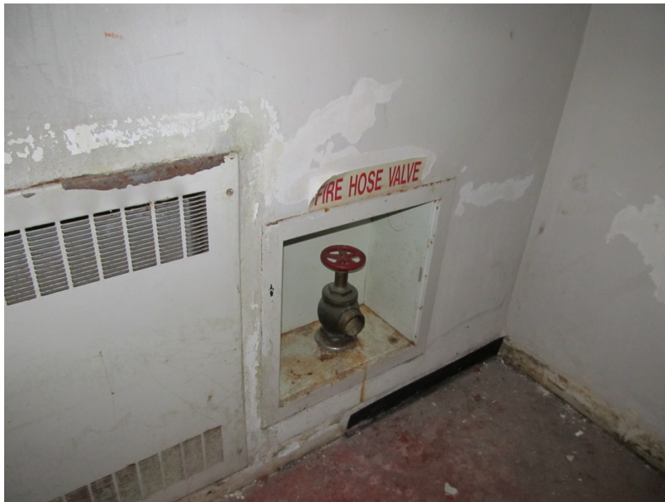
Typical Stairwell Fire Hose Connection
