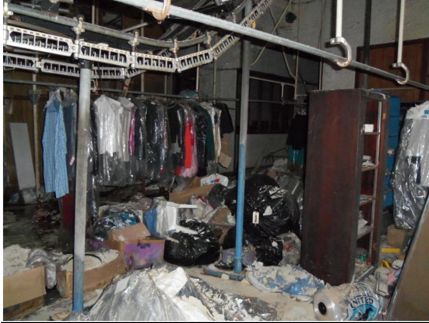
Typical area at first floor.
