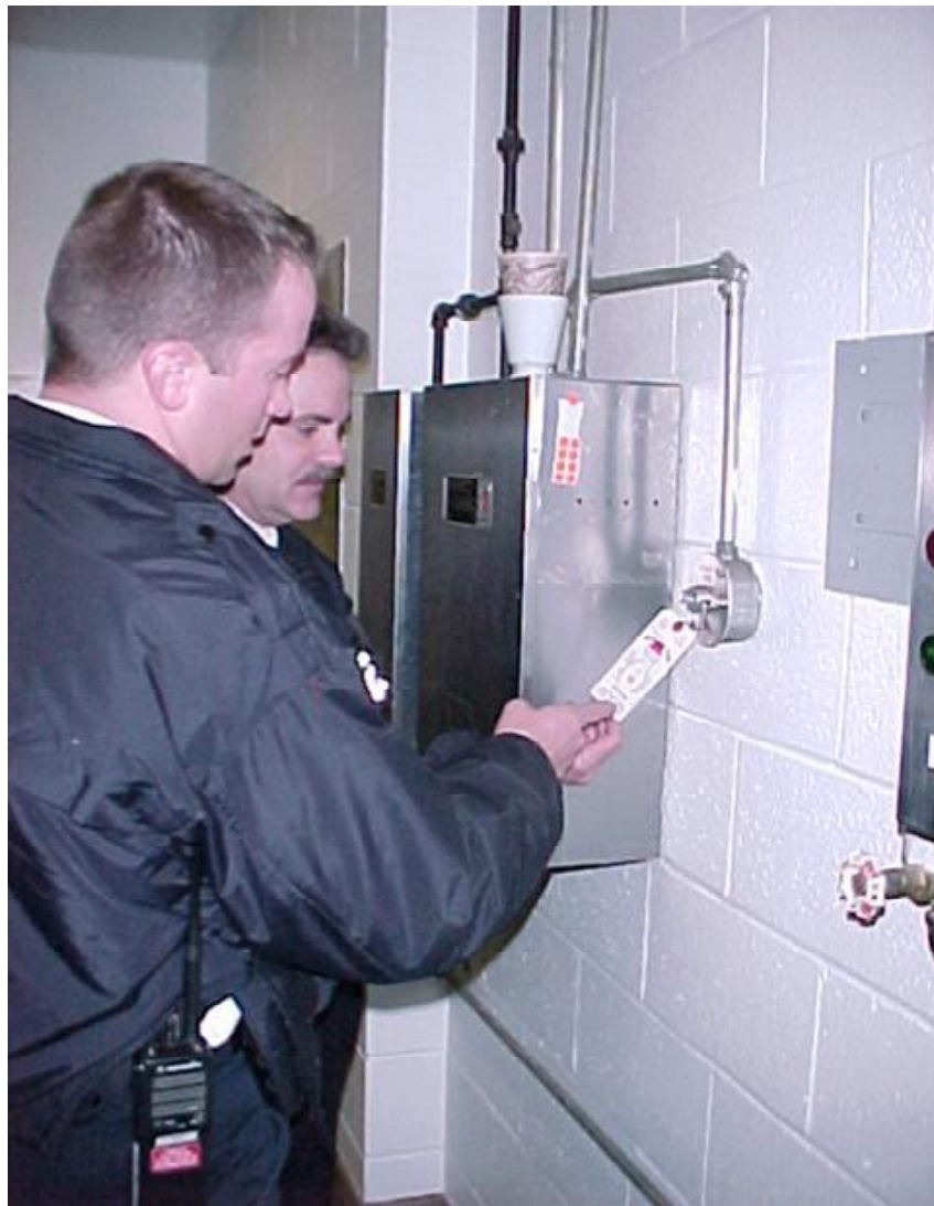
Fire Inspectors Mark Scialdone and Sam Alicata check the expiration date on a fire suppression system control box.
