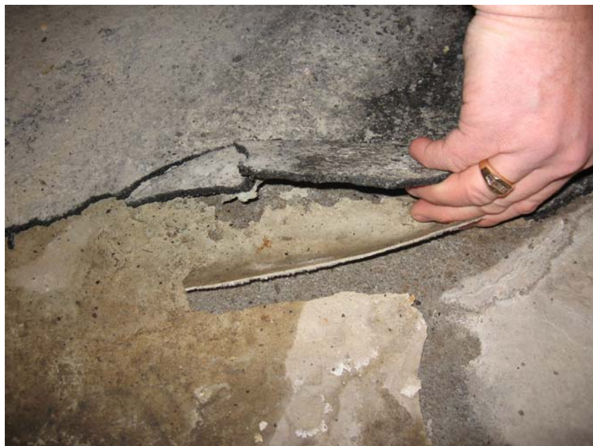
Photo 8 – Aged and Debonded Asphaltic Coating
