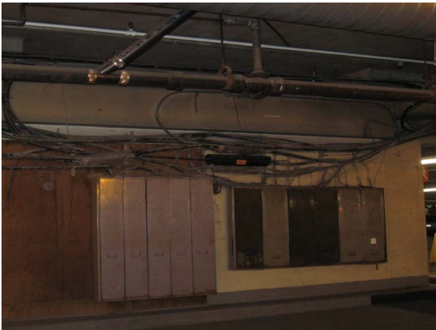
Photo 29 – Main Telephone Cabinets for Garage and Mall
