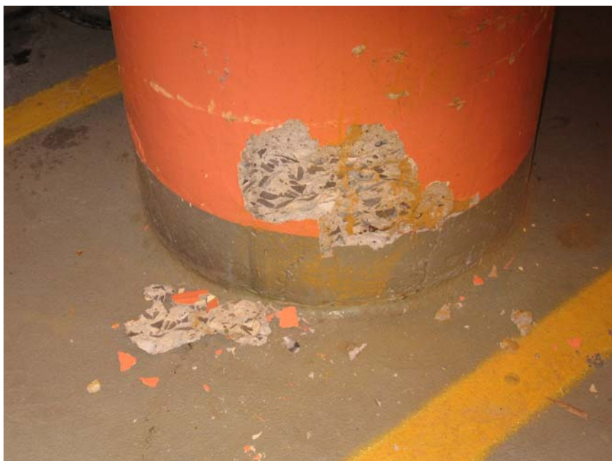
Photo 20 – Column Spall
