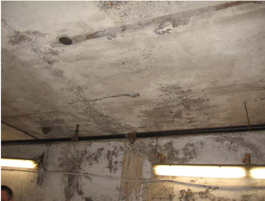
Photo 3 – Ceiling Delamination / Loose Concrete
