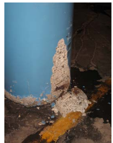
TYPICAL BOTTOM OF COLUMN DETERIORATION ON LEVEL 'C'
