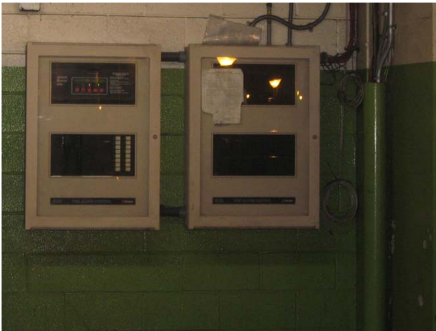
Photo 27 – Main Fire Alarm Panels Located on Level 'A' outside of Escalator Lobby
