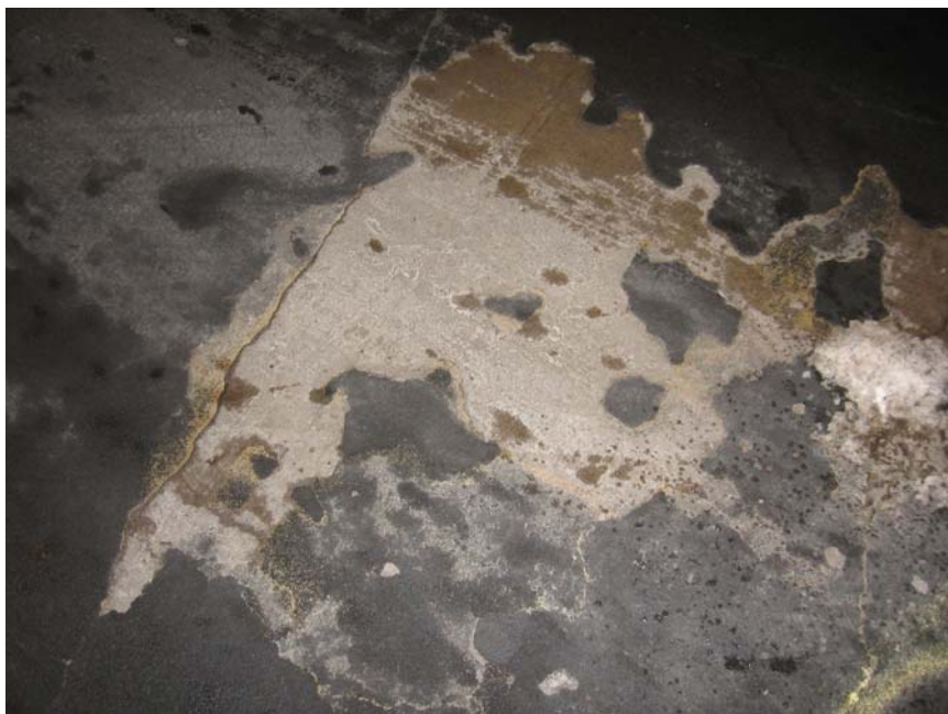
Photo 19 – Debonded / Missing Traffic Topping
