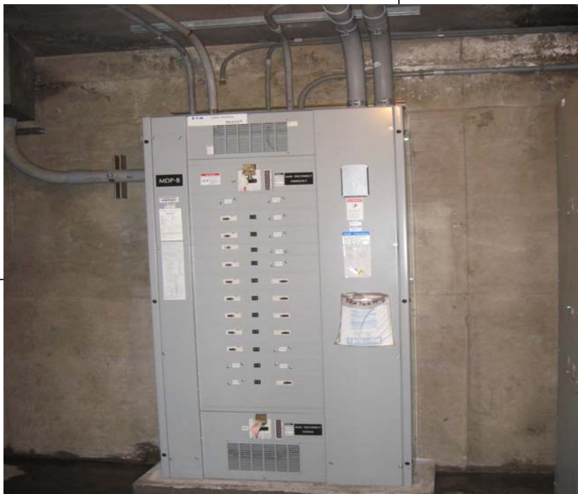
Photo 34 – MDP A in Main Electrical Room on Level 'B' Recently Replaced
