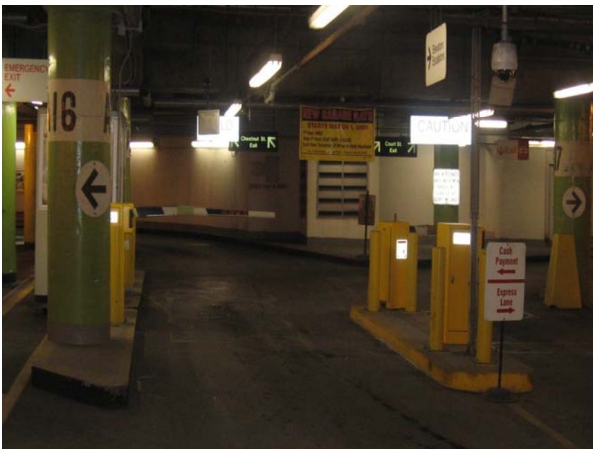
Photo 30 – PARCS Equipment on Level 'B'
