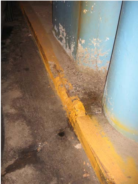
Photo 13 – Deteriorated Curb Face
