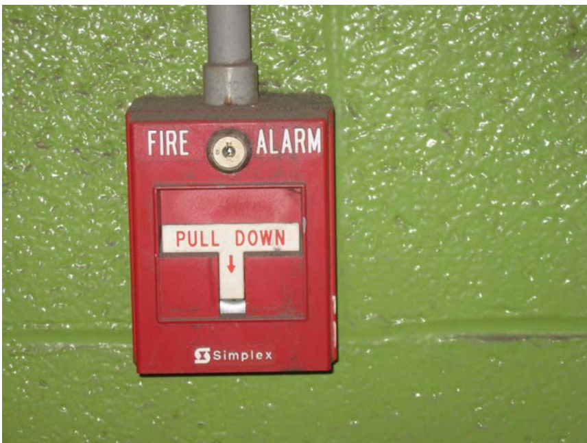
Photo 26 – Typical Fire Alarm system Manual Pull Station
