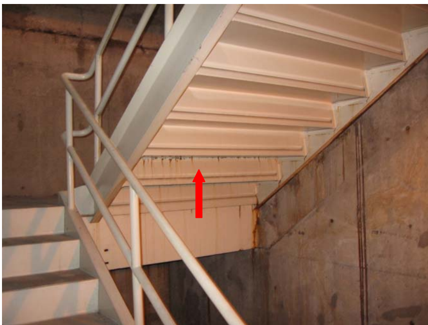
Photo 16 – Stairwell, Note Rust on Bottom of Pan.
