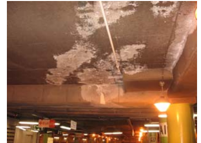
STAINED AND DELAMINATED CEILING
