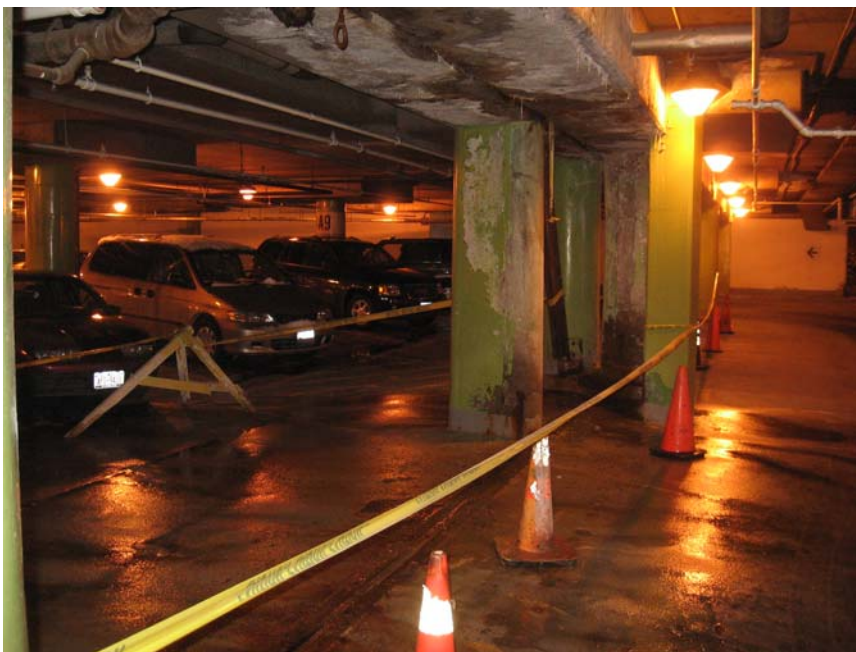
Photo 2 - Severely Deteriorated Beams And Columns Under Leaking Expansion Joint
