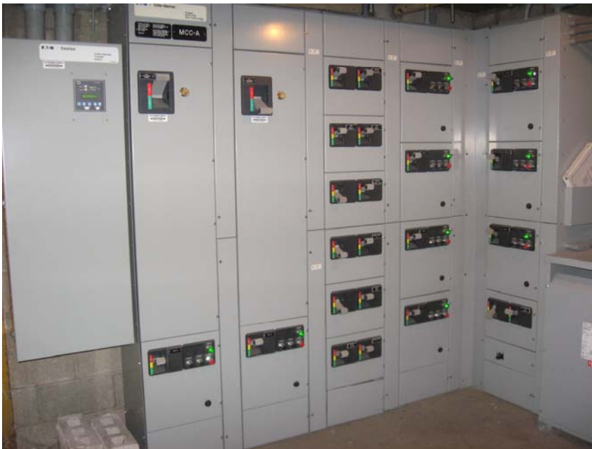
Photo 33 – MCC Electrical Room 204 on Level 'B' Recently Replaced
