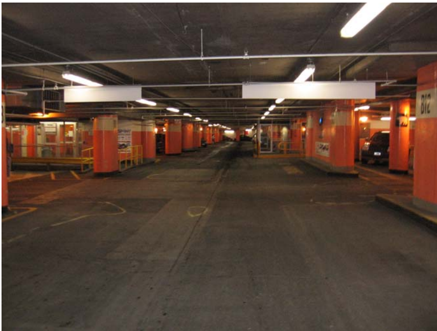
Photo 14 – Main Drive Aisle Area with Asphaltic Coating
