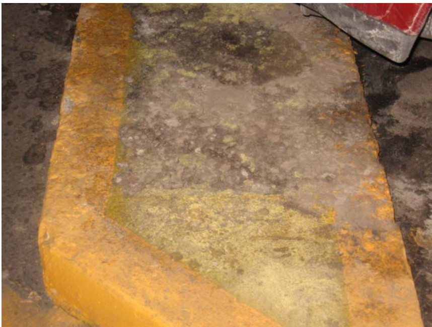
Photo 12 – Curb with Scaled Surface @ Level C
