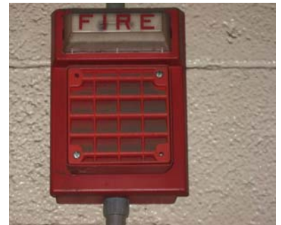
TYPICAL HORN STROBE – THIS DEVICE IS NOT IN COMPLIANCE WITH ADA REQUIREMENTS
