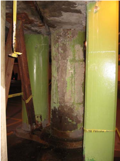
Photo 1 - Severely Deteriorated Beams And Columns Under Leaking Expansion Joint
