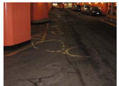
FLOOR DELAMINATIONS PRESENT IN MAIN DRIVE LANE
