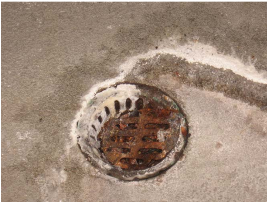
Photo 4 – Broken Drain Grate is Trip Hazard
