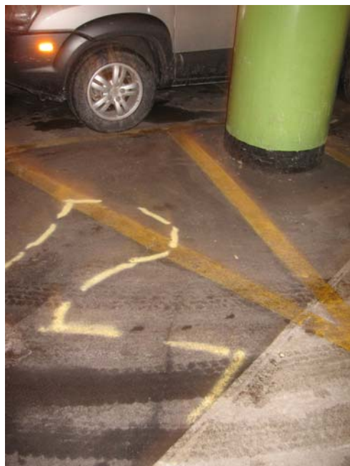
Photo 7 – Outline of Floor Delamination
