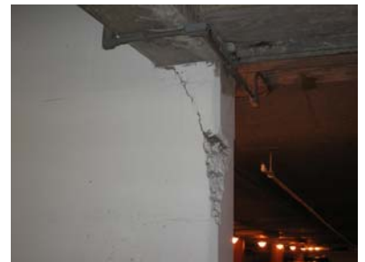
CRACKED END OF WALL COMPROMISING THE BEAM SHEAR BEARING
