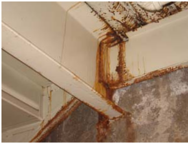
NOTE RUST ON STAIR FRAMING AND UNDER SIDE OF METAL PAN
