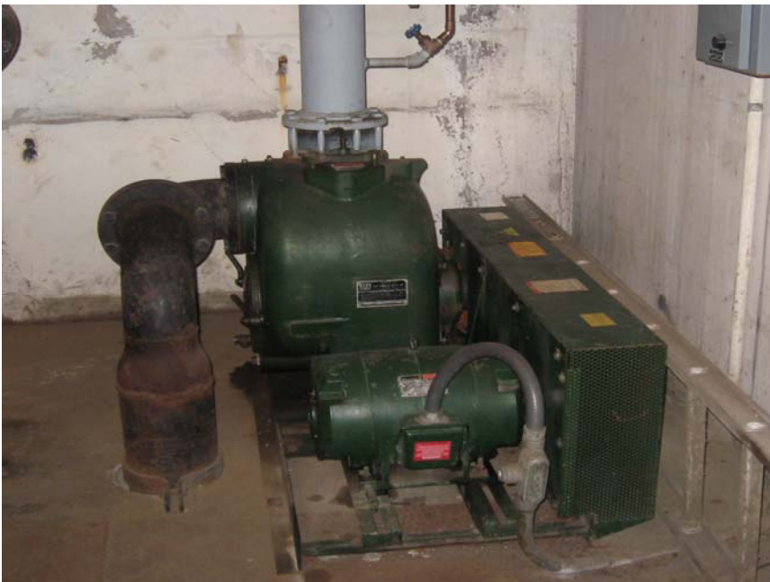
Photo 32 – Sewage Ejector Pump on Level 'C' – One of Two Pumps in this Room
