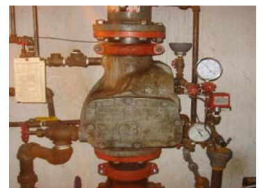
TYPICAL OLD FIRE SPRINKLER MAIN VALVE
