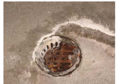
BROKEN FLOOR DRAIN GRATE
