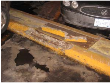
TYPICAL CURB DETERIORATION ON LEVEL C
