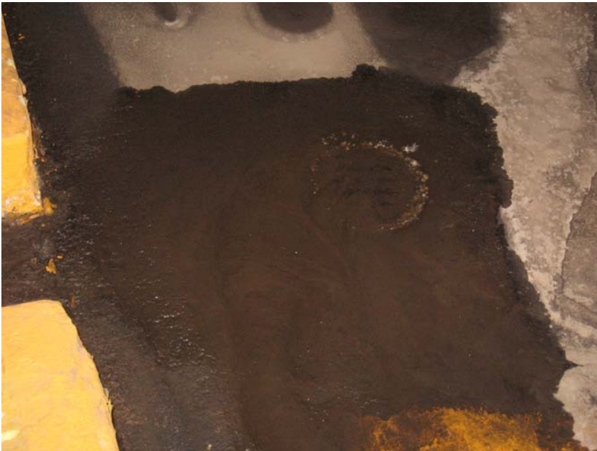
Photo 10 – Plugged Floor Drain Causing Ponded Water
