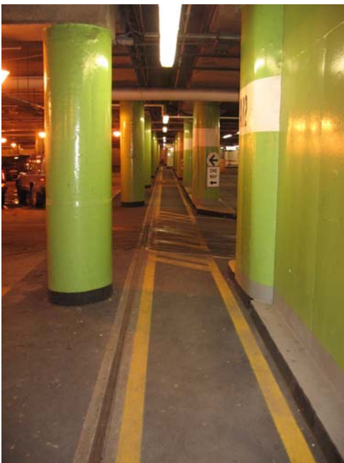
Photo 6 – East/West Expansion Joint
