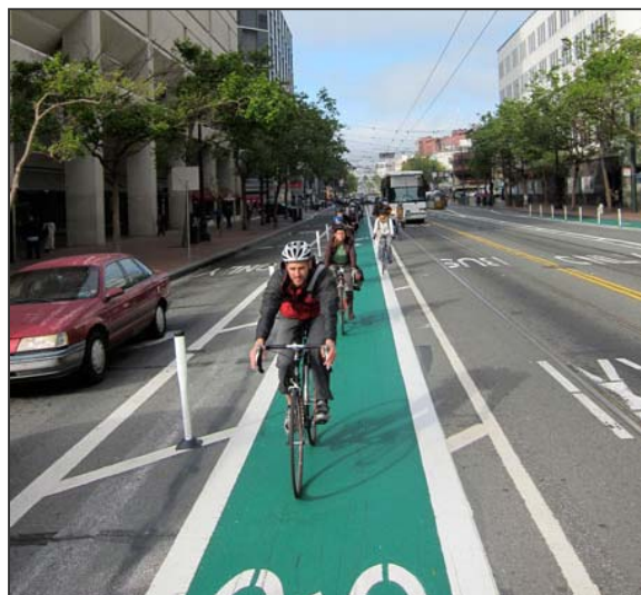
A continuous colored, buffered bike lane treatment in San Francisco, CA (Photo Credit - Matthew Roth)
