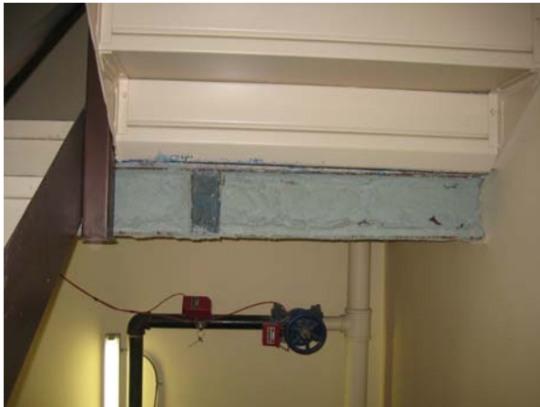
Spray-on fireproofing in stairwell
