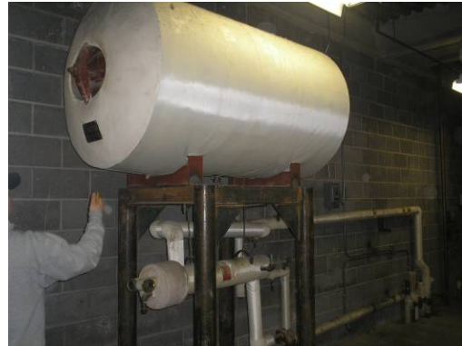
Hot water tank in elevator penthouse
