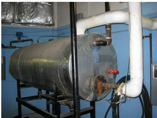
Expansion tank in boiler room
