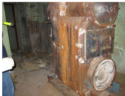
Boiler core in boiler room
