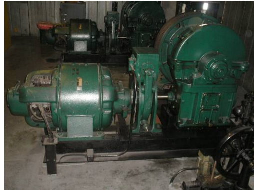
Elevator penthouse motor
