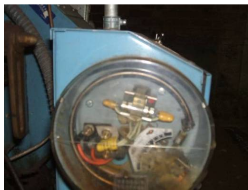
Mercury Switch - McCurdy's sub-basement
