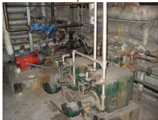
Oil filled vacuum pump in mechanical room
