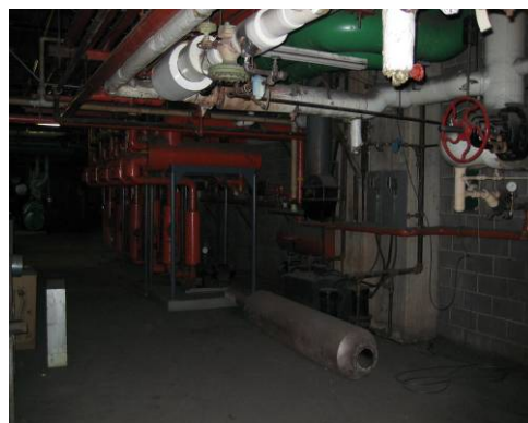
Hot water pumps on southwest wall of mechanical room
