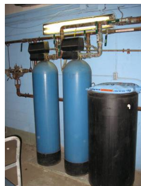
Water softener in Boiler Room
