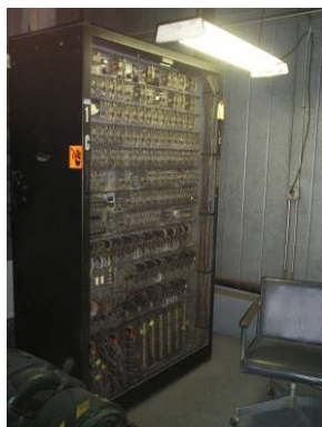
Elevator penthouse panel w/ capacitors
