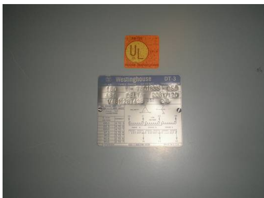
Transformer – dry type, 6 th floor
