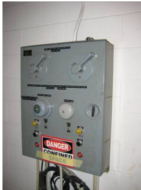
Panel for sump pumps in basement
