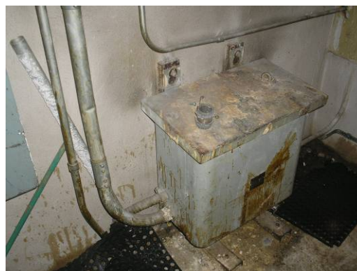
Transformer on 14 th floor
