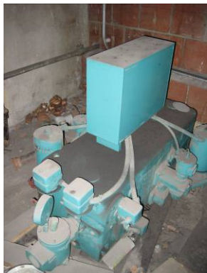
Vacuum pump in back room of basement
