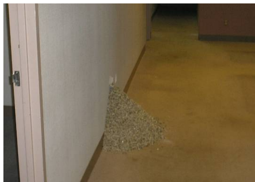
Vermiculite in wall 9 th floor
