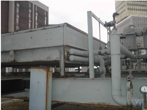
Cooling tower on roof
