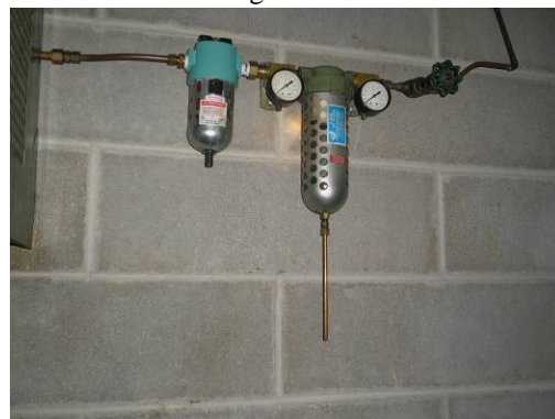
Air line Filter on 7 th Floor
