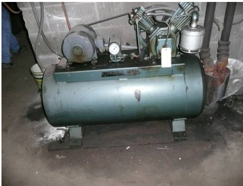
Compressor in sub-basement of McCurdy's Building
