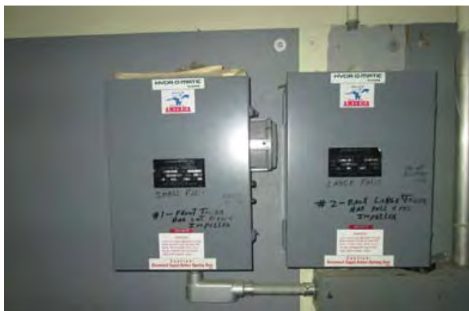
Figure 28 - Pump Controllers
