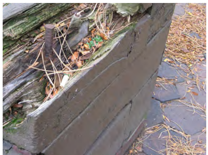
Figure 8 - Timber retaining walls are rotted and deteriorating in many areas.
