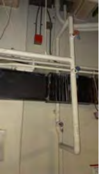
Figure 40 - Line to hose bibb
