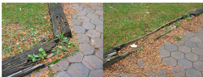
Figure 7 - Timber curbs are rotting and broken in numerous locations.
