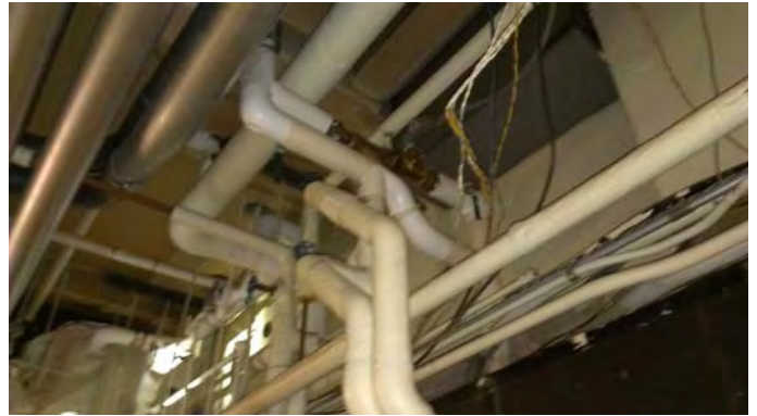
Figure 39 - Fill line with solenoid valve
