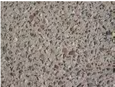
1'-6" Wide Band of Exposed Aggregate Concrete Between Concrete Sidewalk and Curb
