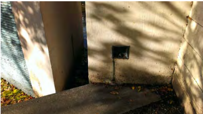
Figure 43 - Wall Hydrant
