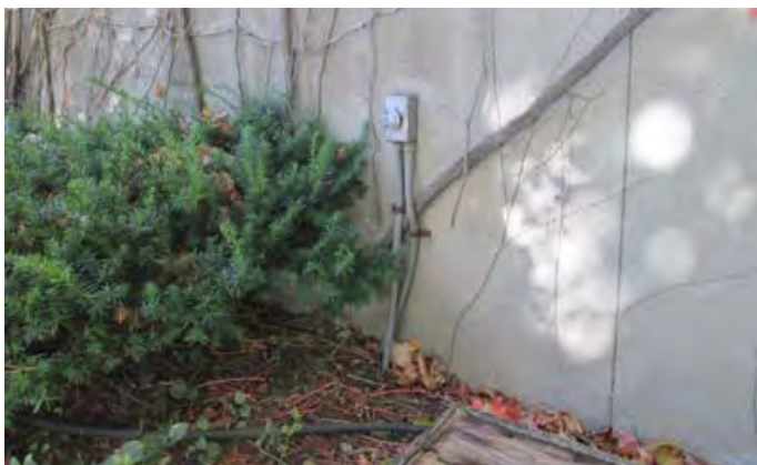
Figure 33 - Receptacle Cover Not Closing Tight
