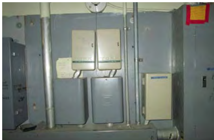
Figure 27 - Time Clocks And Contactors
