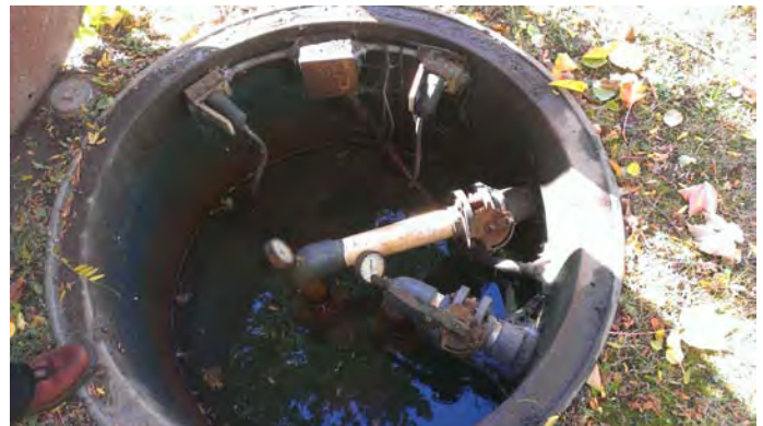
Figure 37 - Water Level and Pump System
