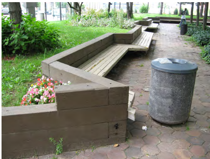
Figure 6 - Existing timber retaining walls and benches.
