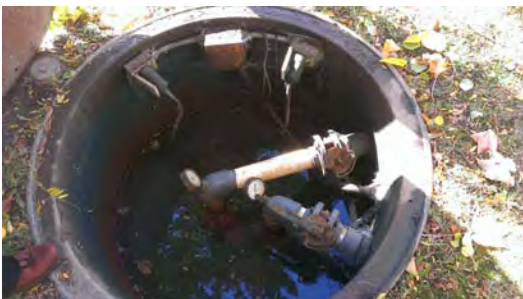
Figure 45 - Level Maintenance Sump Pit
