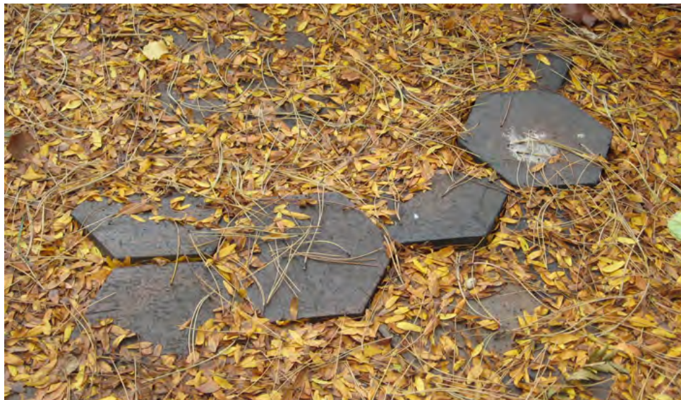
Figure 4 - Hexagonal brick pavers have heaved and become unsafe or are missing in many locations.
