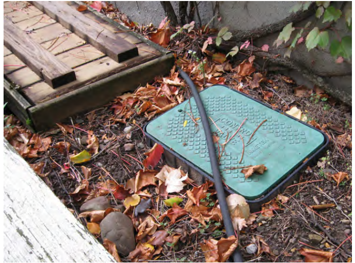
Figure 12 - An existing irrigation system valve box and check-valve hand-hole are located along the north wall behind the retaining wall.
