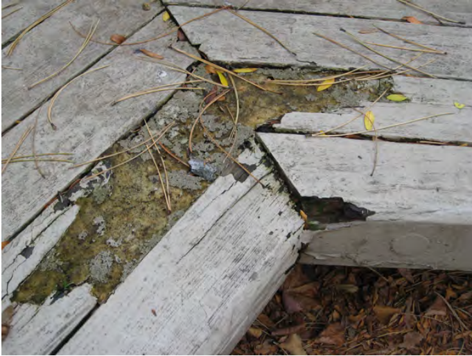
Figure 9 - Damaged and rotting timber benches are at the end of their useful life.
