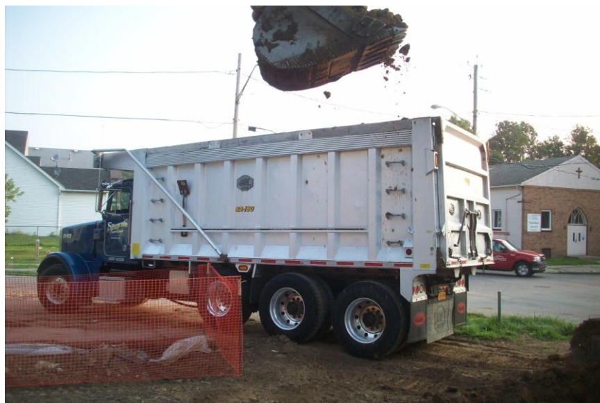
Photo 27 – Direct-loading contaminated soil from Tank 1/Tank 2 Excavation (9/2/2011)
