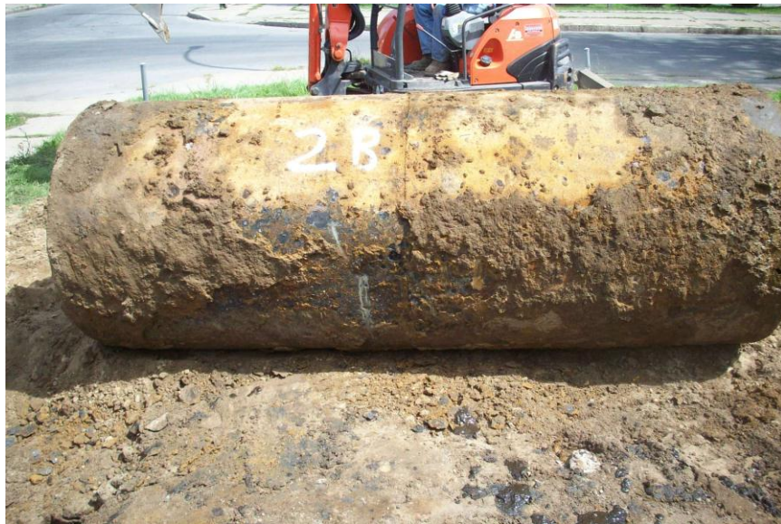
Photo 10– View of the bottom of Tank 2 (8/31/2011)
