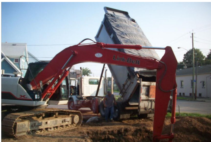
Photo 30 - Backfilling at Tank 1/Tank 2 Excavation (9/2/2011)
