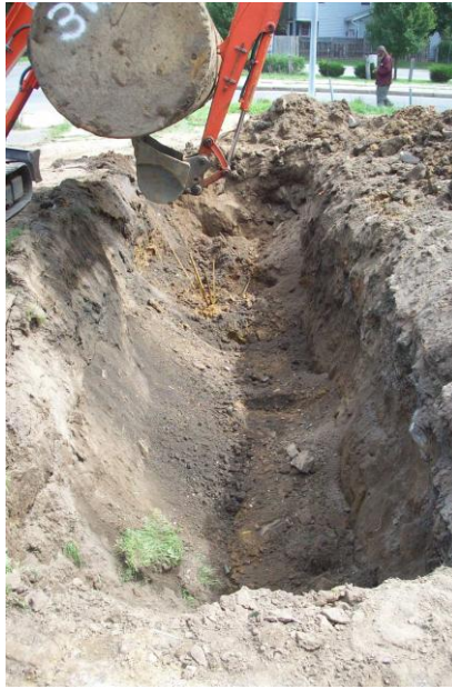
Photo 4– Tank 3 and Tank 4 excavation subsequent to tank removal (8/31/2011)
