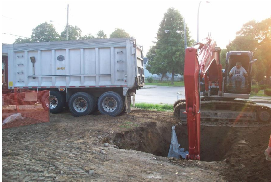
Photo 25 - Soil removal at Tank 1/Tank 2 Excavation (9/2/2011)
