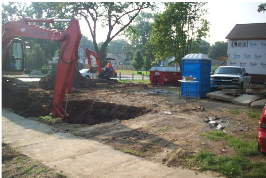
Photo 33 - Soil removal at Tank 3/Tank 4 Excavation (9/2/2011)
