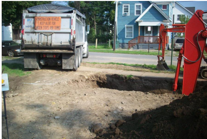
Photo 34 - Soil removal at Tank 3/Tank 4 Excavation (9/2/2011)
