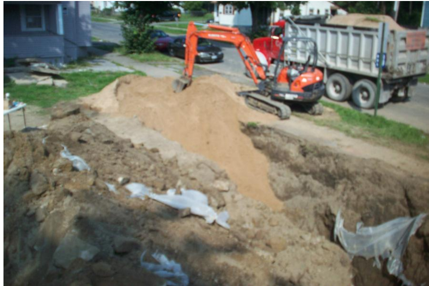
Photo 37 - Backfilling at Tank 3/Tank 4 Excavation (9/2/2011)
