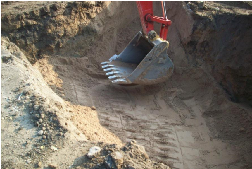
Photo 29 - Backfilling at Tank 1/Tank 2 Excavation (9/2/2011)
