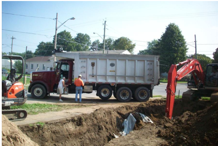
Photo 35 - Soil removal at Tank 3/Tank 4 Excavation (9/2/2011)
