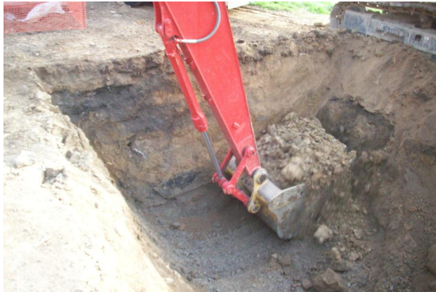
Photo 26 - Soil removal at Tank 1/Tank 2 Excavation (9/2/2011)
