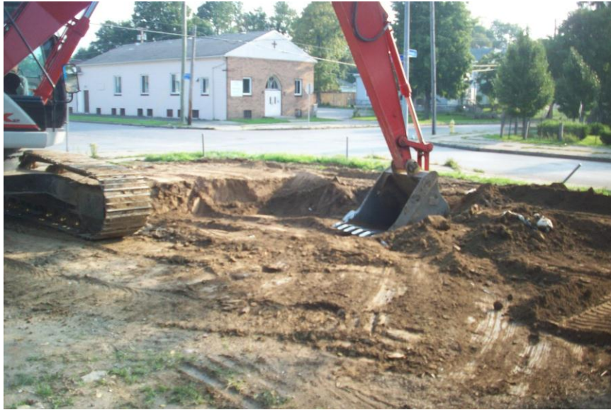
Photo 31 – Backfilling/.compacting at Tank 1/Tank 2 Excavation (9/2/2011)
