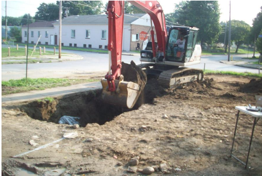
Photo 32 - Soil removal at Tank 3/Tank 4 Excavation (9/2/2011)
