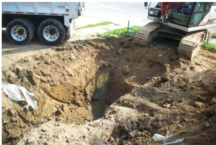
Photo 36 - Soil removal at Tank 3/Tank 4 Excavation (9/2/2011)
