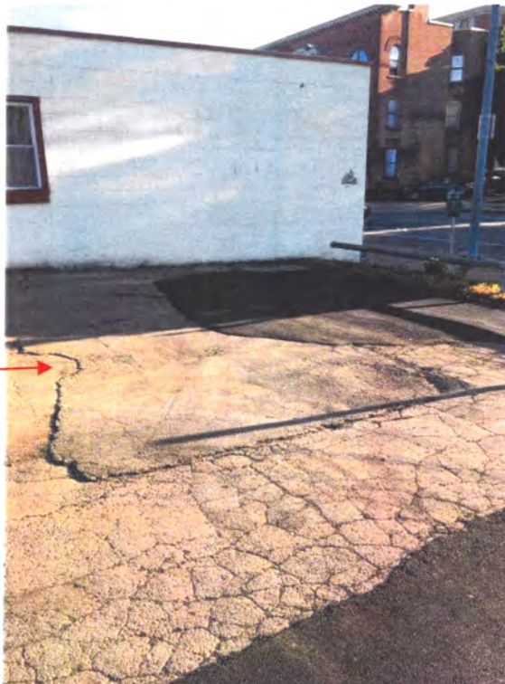
View of an approximate 8' x 12' rectangular-shaped asphalt patch in the parking lot on the northeastern portion of the assessed property, which could be associated with a former UST, looking northeast.
