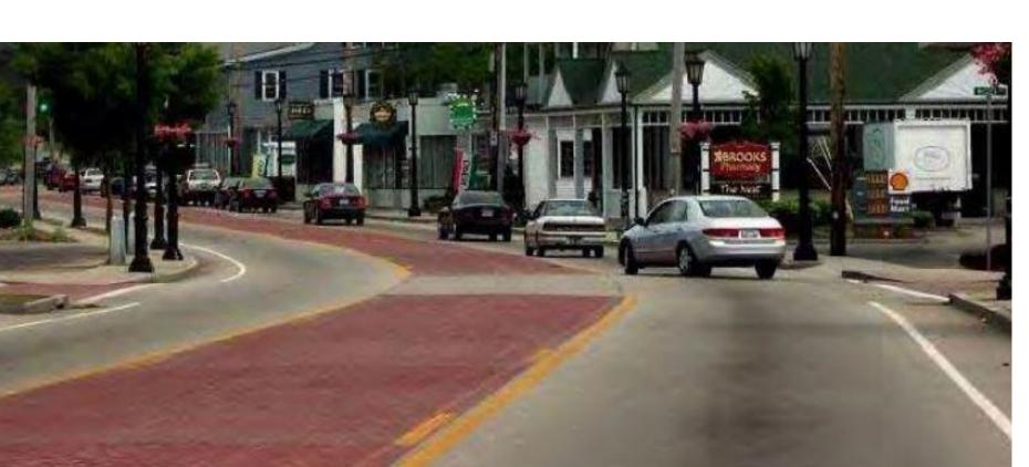
The center two-way leftturn lane will be constructed with a colored surface that contrasts with the asphalt in the travel lanes. While marked and available for use by vehicles, this feature will visually narrow the roadway and promote slower speeds.
