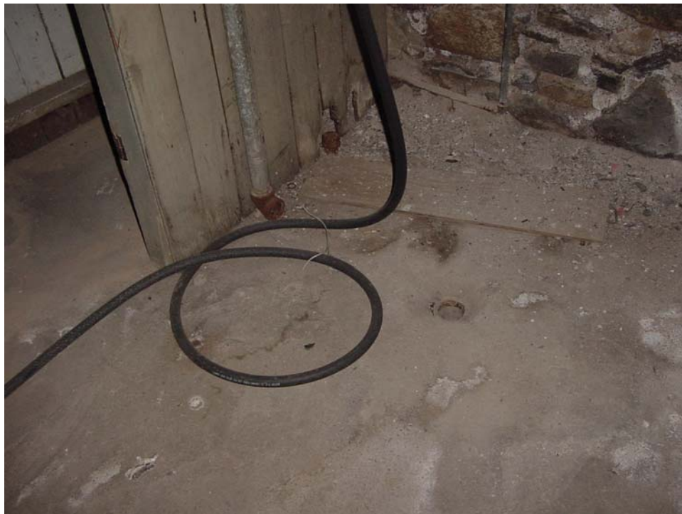
Drain/opening in basement floor.
