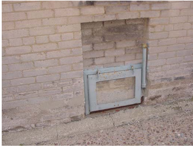
Coal chute and vent.
