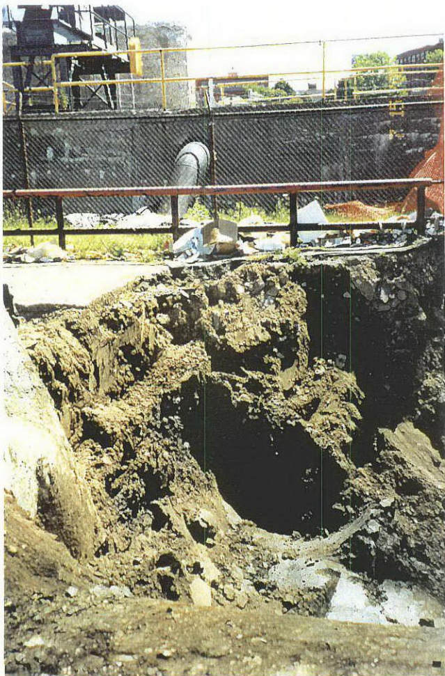
PHOTO 11: SOIL EXCAVATION (440 ft 2 area) North Wall upon removal of 2000-gallon UST
