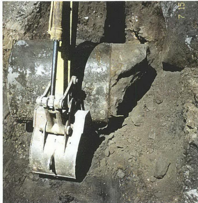
PHOTOS 7 THRU 10: REMOVAL OF 2000-GALLON CLOSED-IN-PLACE UST
