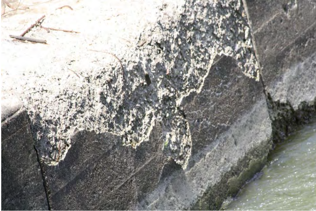
PYLON FOUNDATION CONDITIONS AT WATER LEVEL
