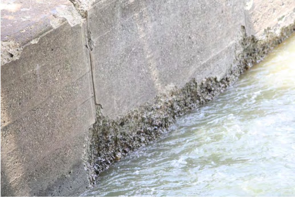
PYLON BASE CONDITIONS AT WATER LEVEL
