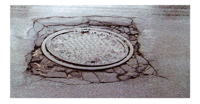
Cancel Collect Submit Manhole MH1234 1406517.48E 1151819.39N depth Pavement Condition \* 0-25: Serious - Failed Corrective Action 2 \* 0-25 Serious - Failed: Mitigate within 30 calendar days - Reconstruct pavement section in kind - Apply tack coat between al... Cover/grate flush with frame? \* Yes Corrective Action 3 \* Yes: No action Overall Structual Condtion \* **Needs Structural Review** Estimated Date of Restoration \* 12/29/1899, 7:00 PM Notes Photo Included? \* \* indicates required field
