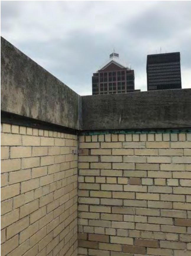
PHOTO 9 S.E.N. Entrance Corner Vertical Joint Separation
