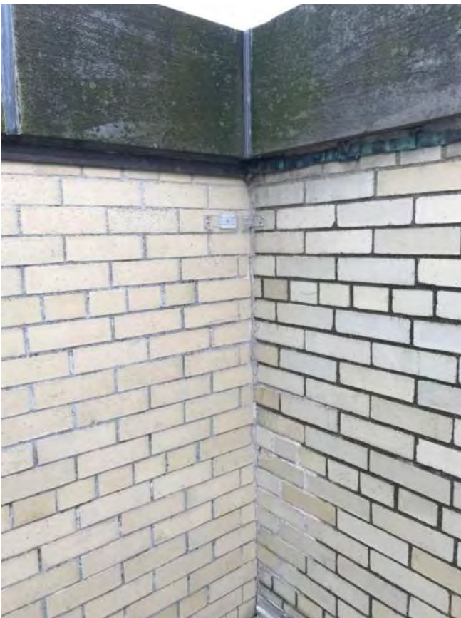
PHOTO 2 S.W. Riverside Corner Mortar Crack
