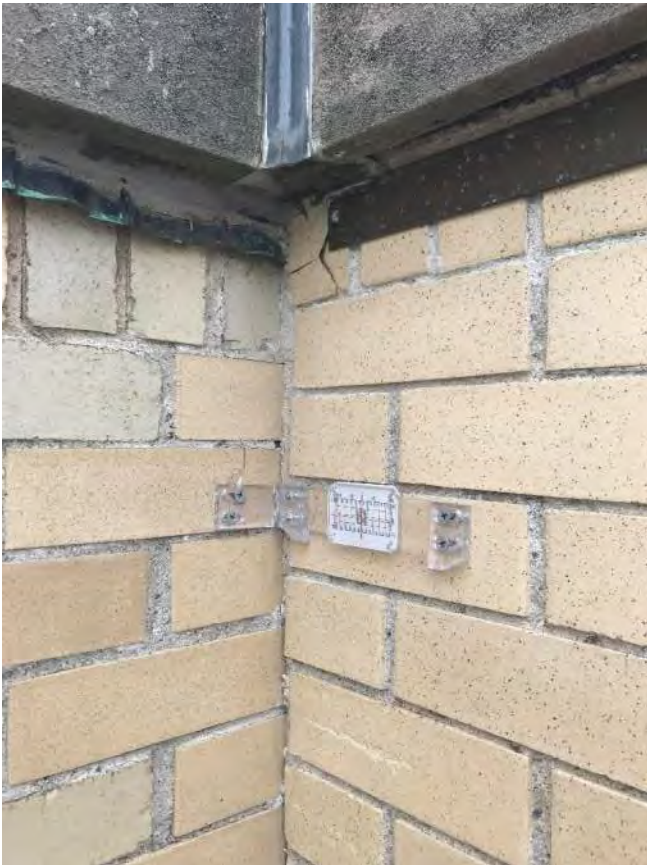
PHOTO 10 N.E.S. Entrance Corner Vertical Joint Separation
