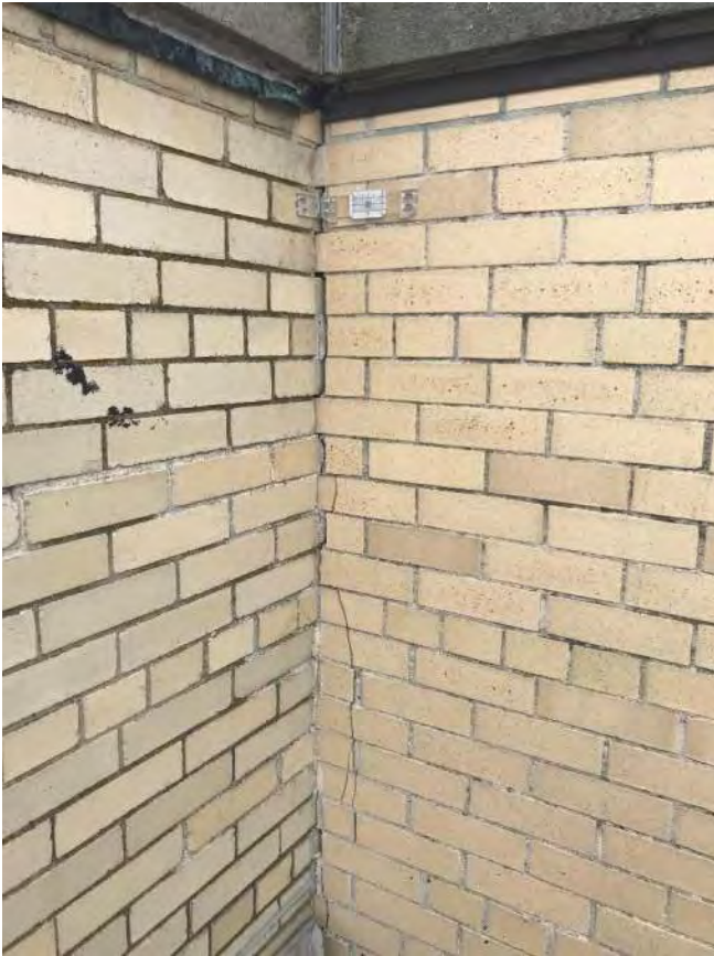
PHOTO 1 N.W. Riverside Corner 3/8" Wall Separation
