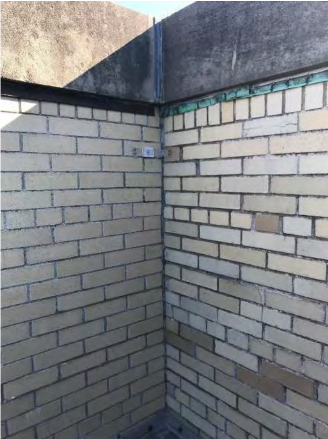
PHOTO 9 S.E.N. Entrance Corner Vertical Joint Separation
