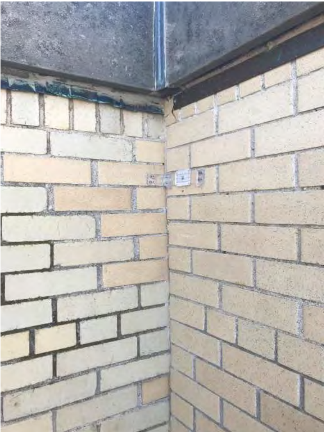
PHOTO 10 N.E.S. Entrance Corner Vertical Joint Separation
