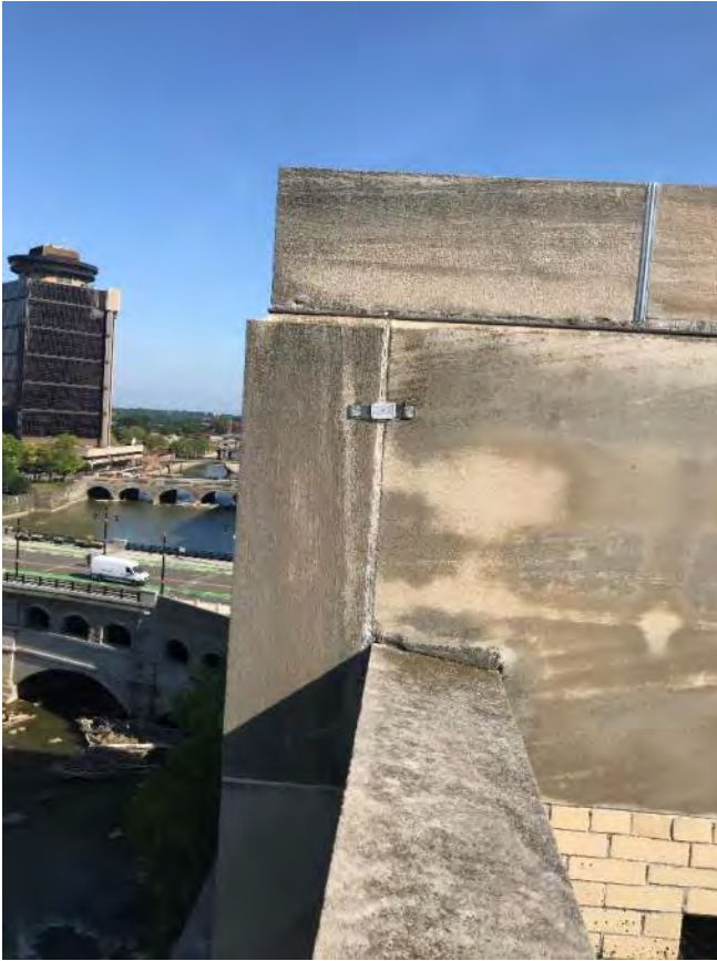
PHOTO 7 S.W. Riverside Exterior Vertical Joint Separation
