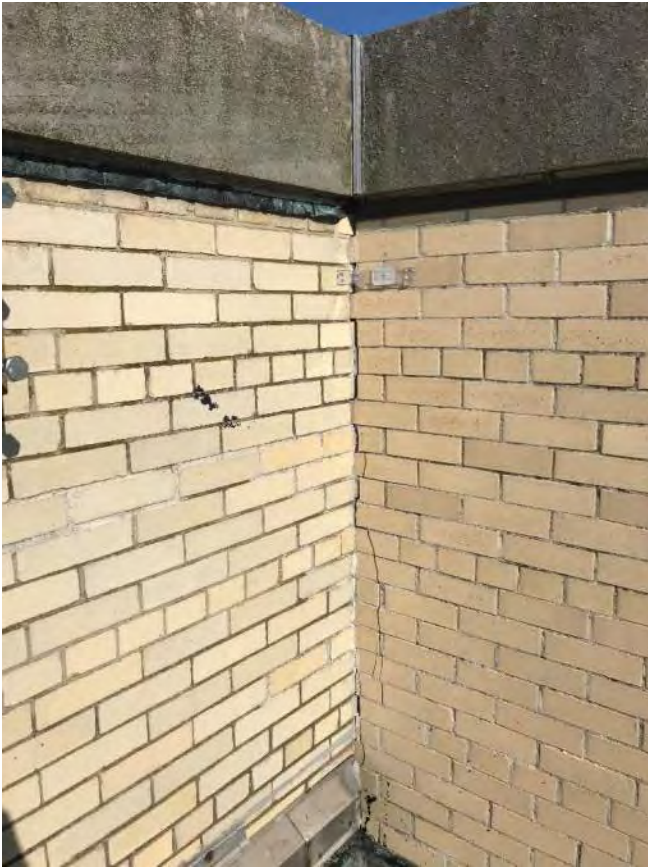
PHOTO 1 N.W. Riverside Corner 3/8" Wall Separation
