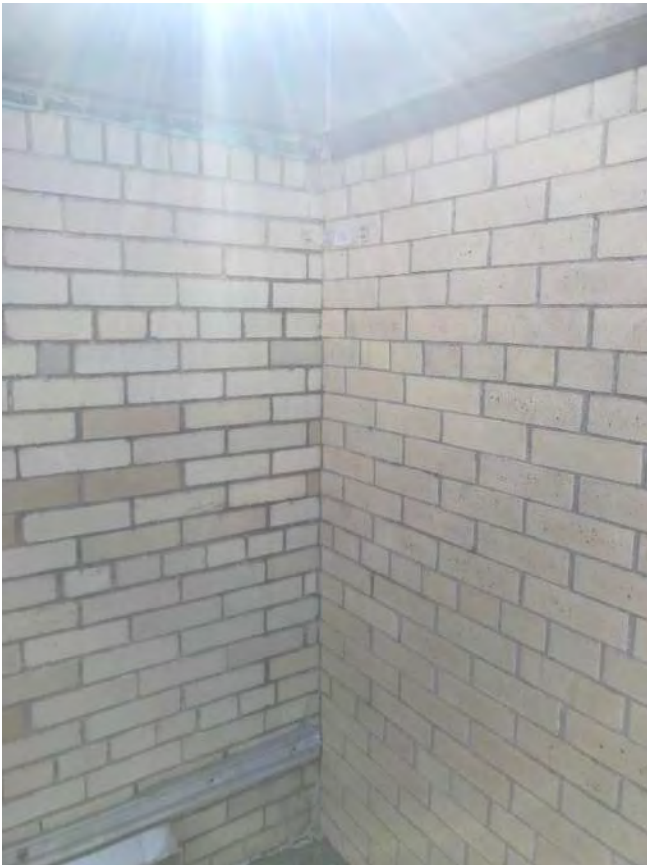
PHOTO 8 S.E.S. Entrance Corner Vertical Joint Separation
