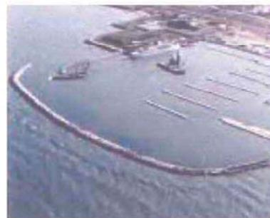
The core of the protective breakwater at the Hammond Marina (Hammond, Ind.) consists of 65,000 tons of ACBF slag. After extensive testing, Indiana's Department of Environmental Management approved ACBF slag as an acceptable product for use in Lake Michigan.
