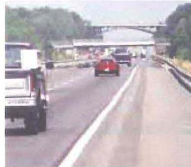
Ohio toll road: ACBF slag was utilized in asphaltic wearing course for superior friction properties.
