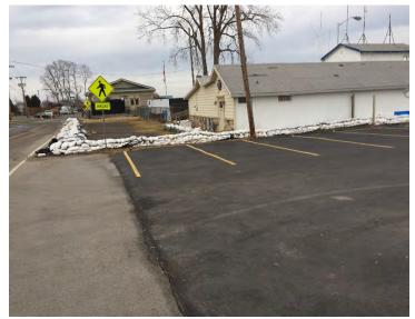
**Figure 2-11** U.S. Coast Guard Auxiliary Shown with Sand Bag Dike to Protect Against Flooding
