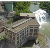
**#7 View of hydro plant** – This building houses three turbines, which together generate 46 MegaWatts of electricity, enough to power over 30,000 homes. Known as Station 5, this hydro plant began operating in 1917. To reach the turbines, water flows down a 2,000-foot-long tunnel. The tunnel begins upstream, at a rack house above the Middle Falls, which you'll see later in this tour.
