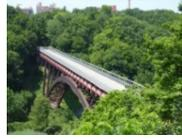
**#2 Clean Waters Bridge**- The bridge was built to hide two 6-foot-diameter pipes which bring excess wastewater from the west side of the river to a treatment plant in on the east side. Built in 1985, the twin arch ribs are 80 feet tall. Ramps and stairs provide safe pedestrian access to the bridge.
