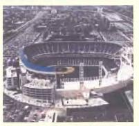
The new Comiskey Park (Chicago, IL) contains over 900,000 lightweight concrete block, used EXPANDED BLAST FURNACE SLAG AGGREGATE in order to achieve the desired weight, as well as fire resistance requirements.
