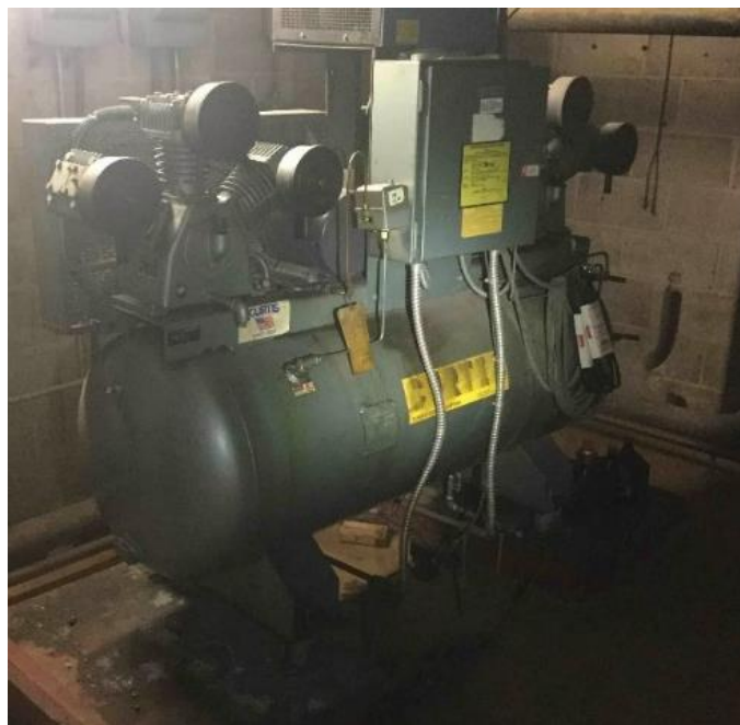
Compressor for Pneumatic Controls System
