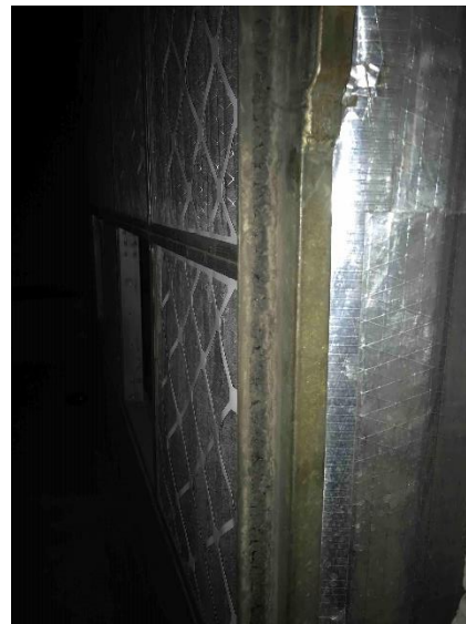
Gaskets at AHU-3 access door
