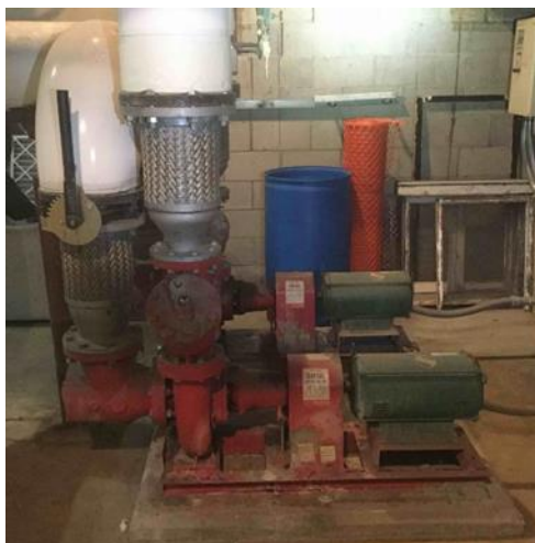
Heating Water Pumps
