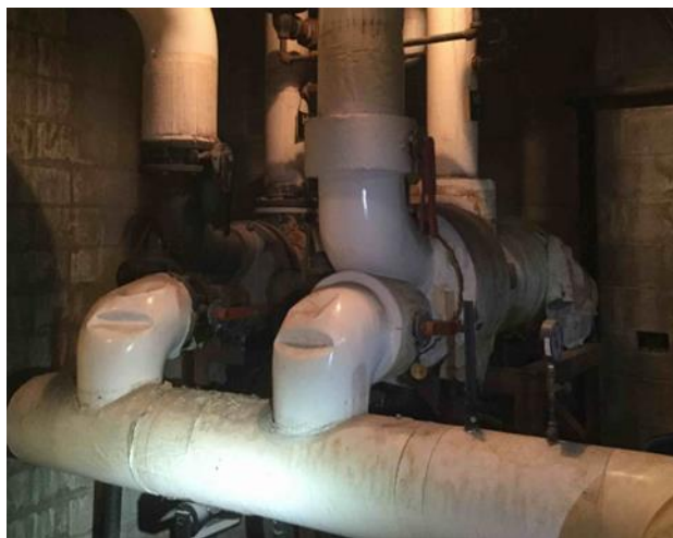
Shell & Tube Heat Exchangers
