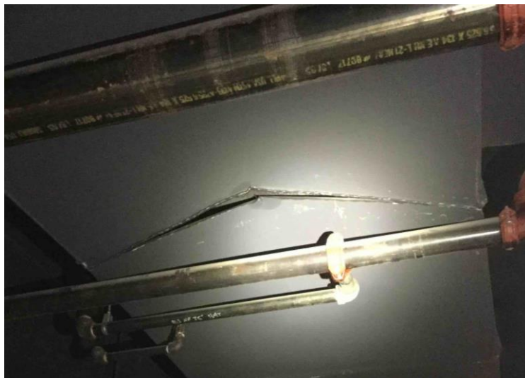
AHU-3 Collapsed Return Air Ductwork
