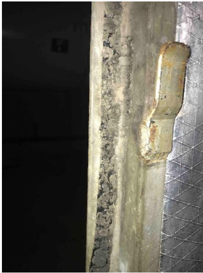
Gaskets at AHU-4 access door
