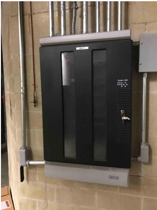
DDC Panel for AHU-5
