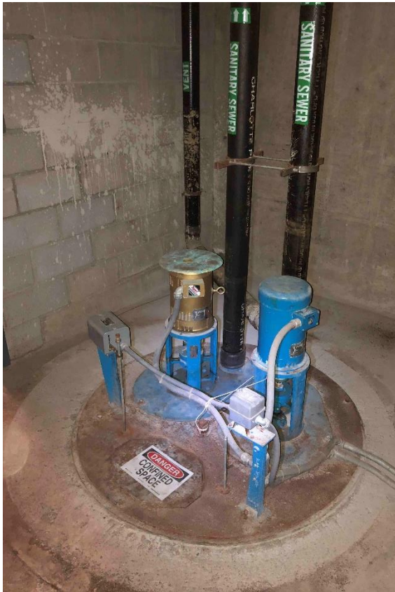
Ejector Pump Station in SE quadrant
