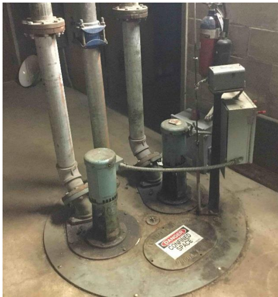
Ejector Pump Station in Water Service Room
