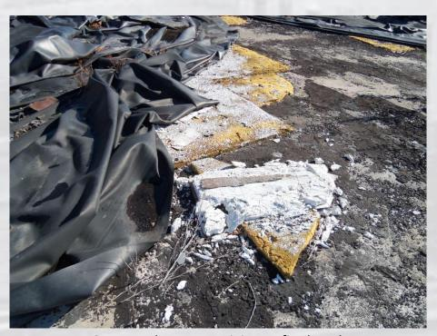
Suspect asbestos containing roofing board
