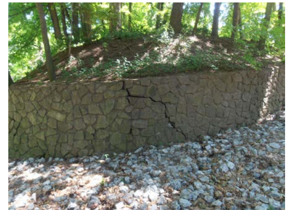
Cracking at Retaining Wall
