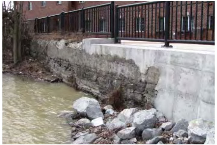
Figure 4-3. Remnant of the Old State dam wall built into the Riverwalk retaining wall behind the new hotel. Photo by CRJA.
